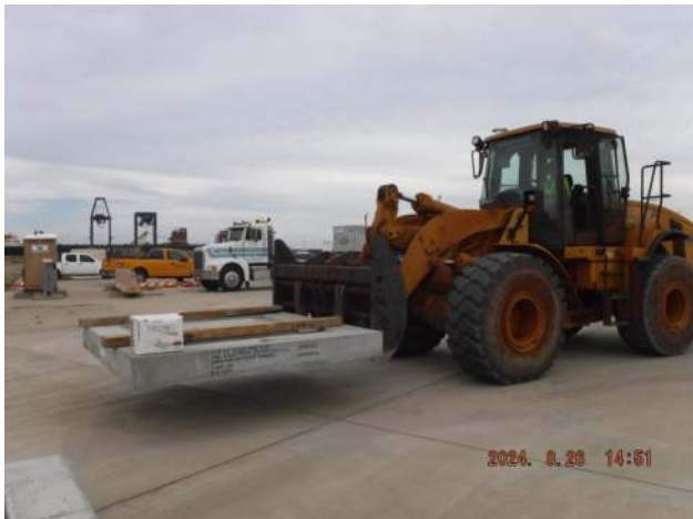
Pier 41: PECL crew unloaded the manhole base
