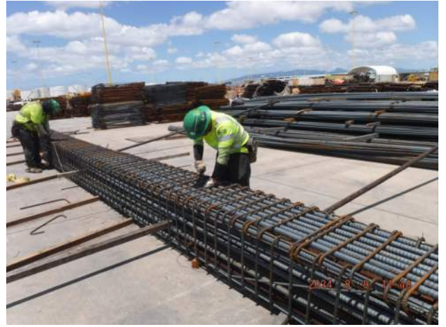
PCCP: HRSPI crew continued to fabricate the tie beam rebar cages
