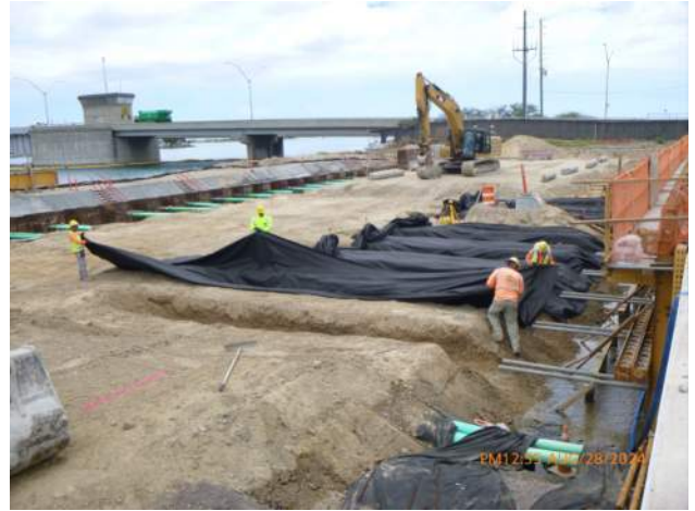
KIWC setting filter fabric in the tie rod trenches on pier 43.
