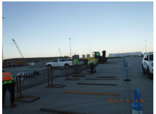
PCCP: HRSPI crew fabricating rebar cage for the tie beams
