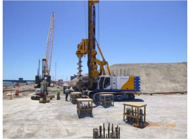
PF drilling for soil mixing around CIDH shafts.
