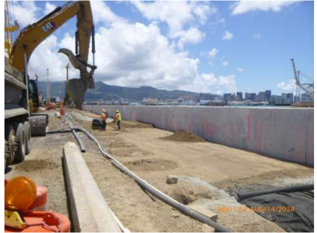
KIWC backfilling on the landside of capping beam pours #21 and 22.
