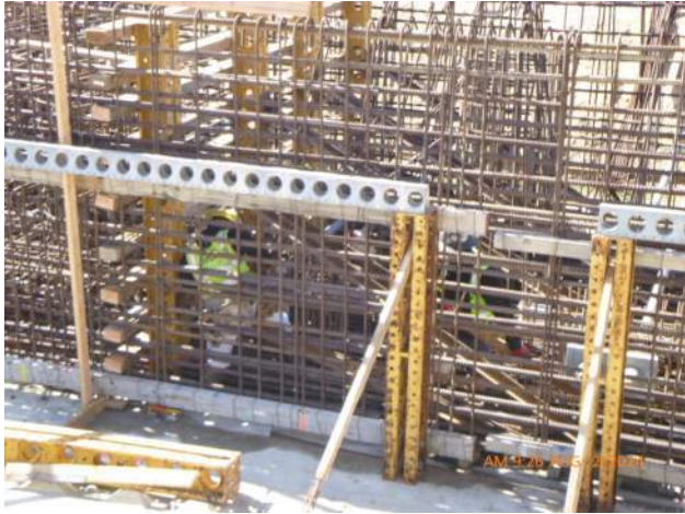
KIWC installing formwork for bulkhead between LSCRB pours #7 and 8.
