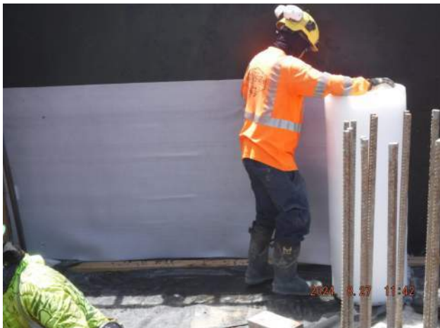
Pier 42: KIWC mason crew installed the "Deck - O- Form" expansion board
