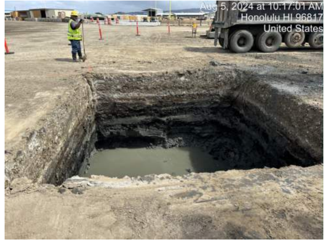
View of the excavation for MH-5A on Pier 42
