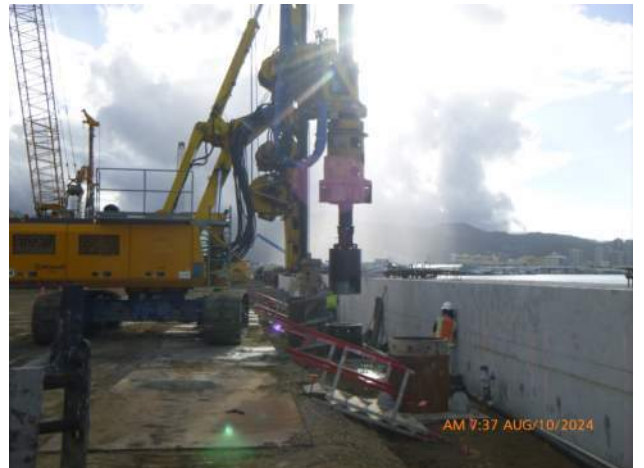
KIWC cleaning out shaft 14-A2S-36.
