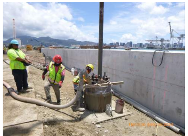
KIWC pouring concrete into CIDH shaft 18-A2S-36.
