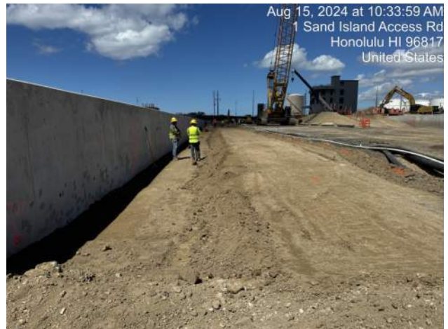
KIWC backfilling lift 3 of the cap beam from P19 to P21
