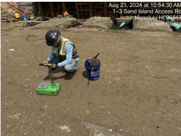
MPE testing lift 2 over the tie rod backfill area on Pier 43
