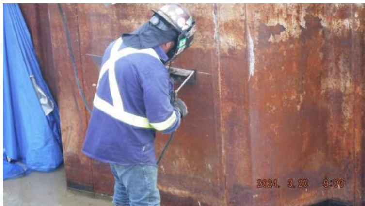
Pier 43: KIWC welder continued to weld the waler braces for P23 of the CWCB
