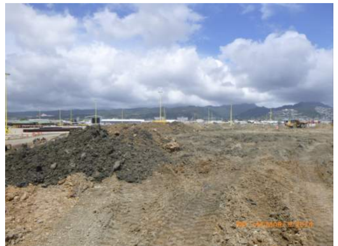
KIWC spreading material over the surcharge area.
