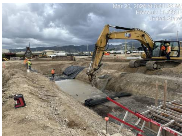
KIWC installing HP 370 fabric on the bottom of the stabilization layer for TD-3 P7
