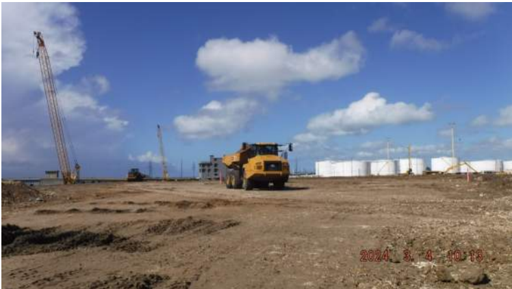
Snug Harbor: KIWC civil crew continued placing the dredged material on the perimeter of the surcharge fill
