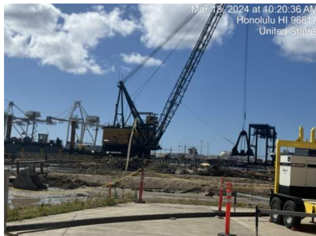
KIWC continued in-water dredging on the corner of Pier 42
