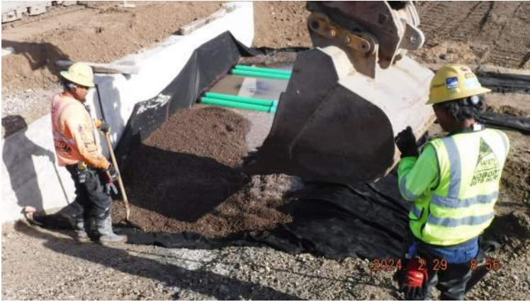
Pier 41: PO Deadman extension - KIWC (Sanu's) placed #3B fine gravel over "burrito" wrapped tie rods
