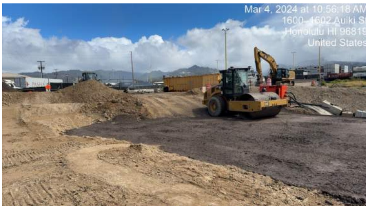
KIWC performing method compaction for backfill lift 7 of the P0 deadman
