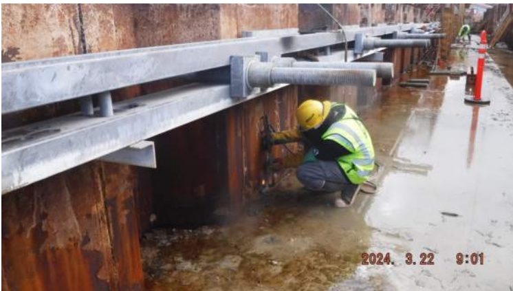
Pier 43: KIWC Bridge and Marine crew continued to burn the holes for the tie rod and rebar penetrations of P17 of the CWCB (STA 6+10.74 to STA 7+03)
