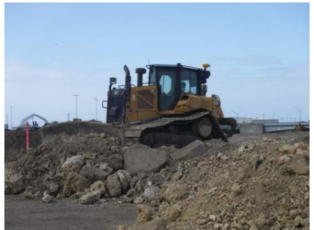
Snug Harbor: KIWC used the CAT D6 dozer to spread the fill material in 12-inch loose lifts for the 13th layer
