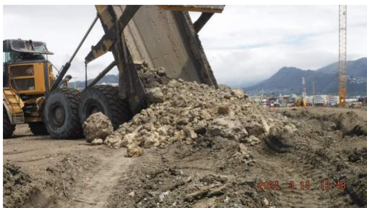
Snug Harbor: KIWC civil crew continued placing the dredged material for the 12th lifts over the surcharge fill
