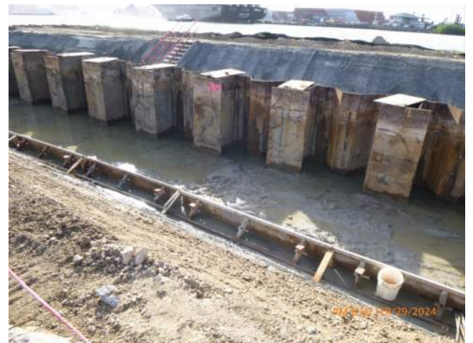
03/29/2024 View of mud mat formwork along the combi wall on pier 43.
