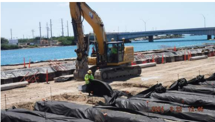
Pier 43 Between P2 and P3 of the LSCRB - KIWC civil crew extended the tie rod trench excavation to 15-feet long
