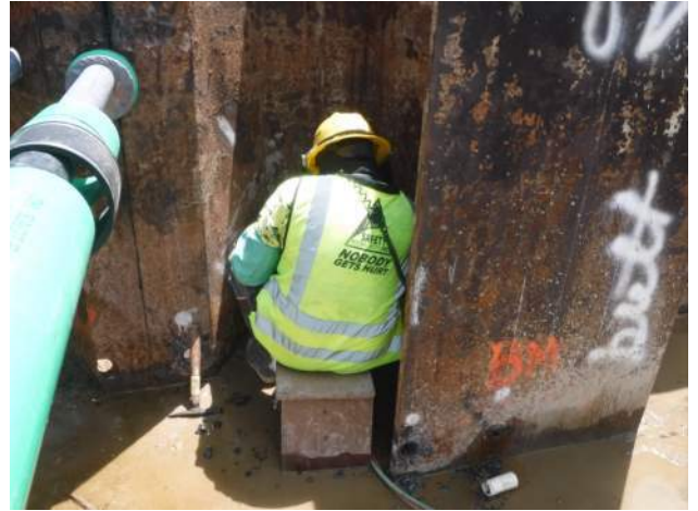
Pier 43: KIWC Bridge and Marine crew continued to lay out and burn holes for the tie rod and rebar penetrations in P17 of the CWCB
