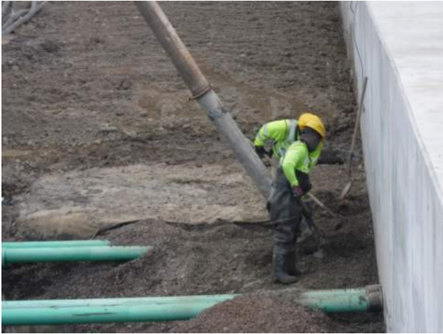
Pier 42: KIWC civil crew used the Vac Truck to remove dredged slurry from the land side of the CWCB on P7 and P8 (Approx STA 13+43 to STA 14+71)
