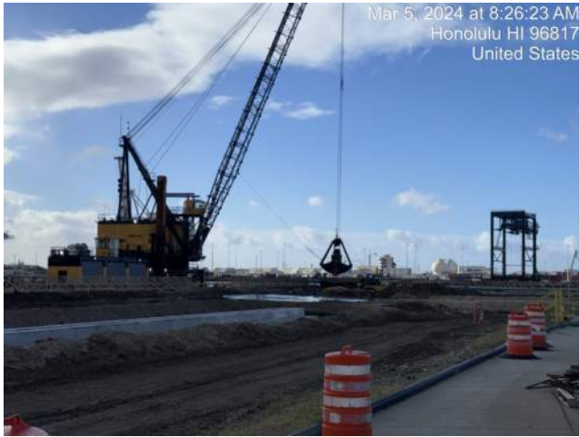
Mar 5, 2024 at 8:26:23 AM Honolulu HI 96817 United States KIWC continued in-water dredging on the corner of P41/42
