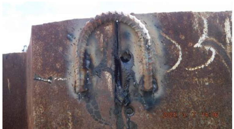
Pier 43: KIWC welding crew weld the "U" rebar between the sheet pile interlock on P21 to P22 of the CWCB (STA 2+83.56 to STA 3+82.64)
