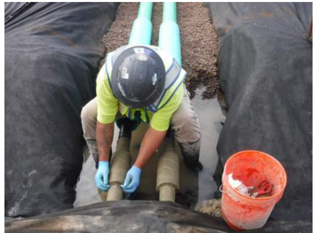
Pier 43: KIWC civil crew (Sanu's) wrapped the tie rod coupler with the Densyl tape followed by the black PVC tape (P2/P3 LSCRB)
