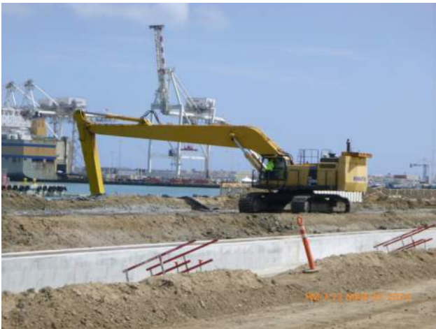
KIWC probing harbor floor using the Cat 1250 excavator.
