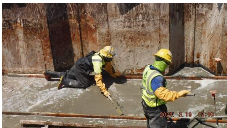
Pier 43: KIWC carpentry placed concrete mixed for the mud mat of P19 on the ocean side of the CWCB
