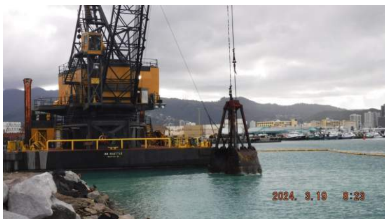
Pier 42: KIWC DB Seattle continued in water dredging from STA 17+00 to 17+75
