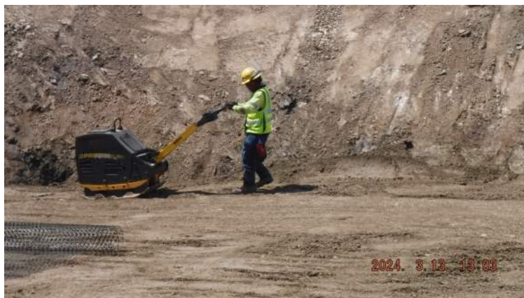
Snug Harbor: KIWC civil crew used the Bomag vibratory steel plate to compact the first lift of the fill placement of the MSE wall
