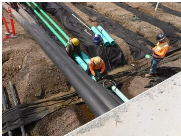
Pier 43: KIWC civil crew (Sanu's) continued to excavate th tie rod trench and installed the tie rod assemblies
