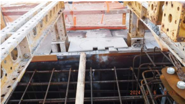
Pier 42: The carpentry crew (Philip's) installed additional form ties and the construction joint board of P14 of the CWCB (STA 8+59.74)
