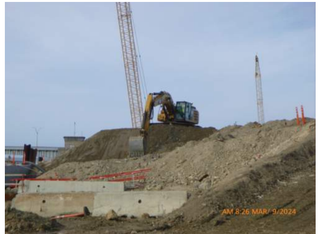
KIWC spreading material over the surcharge area.
