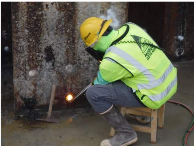
Pier 43: KIWC Bridge and Marine crew continued to burn the holes for the tie rod and rebar penetrations of the CWCB on P 17
