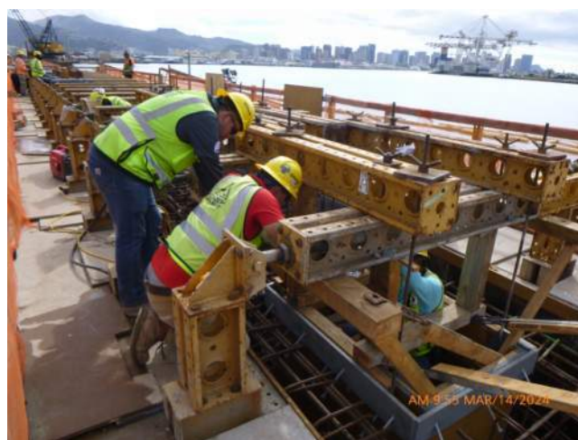
KIWC adjusting ladder rungs in the pour 14 water utility vault.
