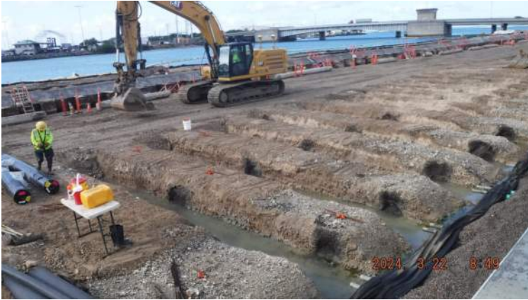
Pier 43: KIWC civil crew (Sanu's) installed the Mirafi geofilter fabric over the tie rod trench excavation between P2 and P3 of the LSCRB
