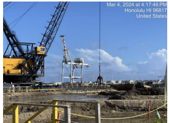
KIWC continued in-water dredging on the corner of P41/42
