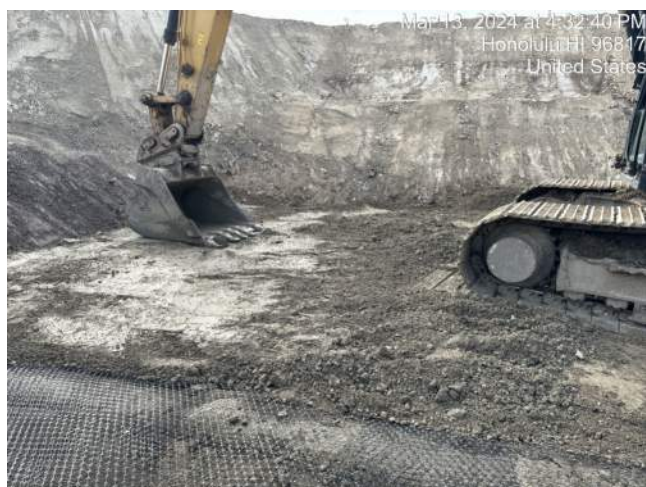
KIWC placing material in the southeast corner of the surcharge
