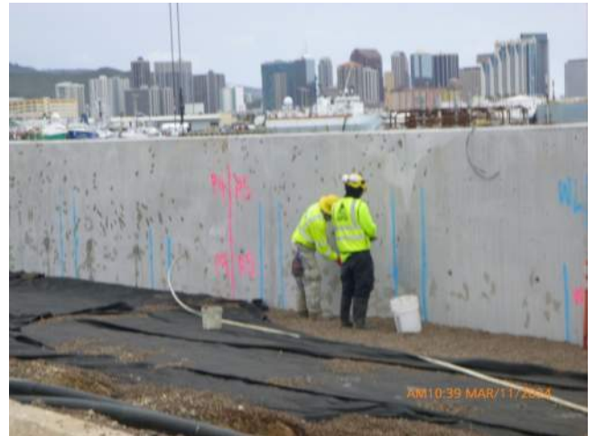
KIWC dy finishing the landside surface of the capping beam.
