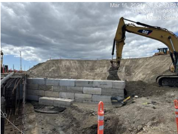
KIWC placing lift 6 of the eco block wall area of Snug Harbor
