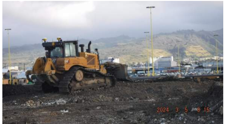
Snug Harbor: KIWC civil used the CAT D6 dozer to spread the fill in 12-inch loose lifts for the surcharge fill
