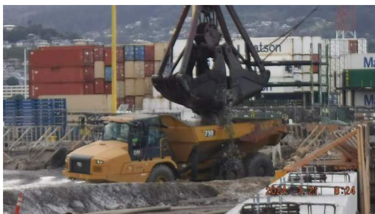
Pier 42: KIWC DB Seattle unloaded the dredged material into the CAT 730 rock truck bed
