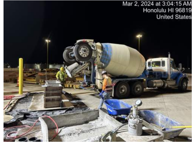
MPE performing concrete testing for truck 1 of the PCCP pours for "H1 blackout"
