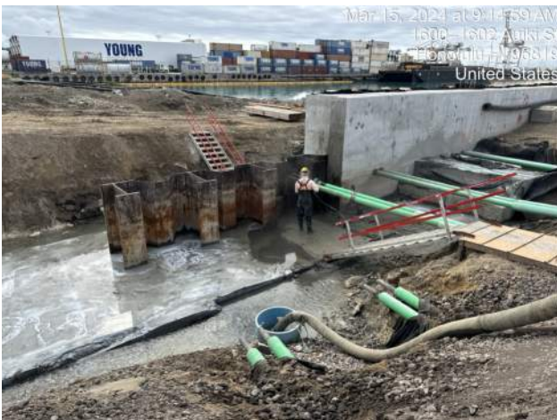
KIWC pressure washing the combi wall at P1 of the combi wall at Pier 41
