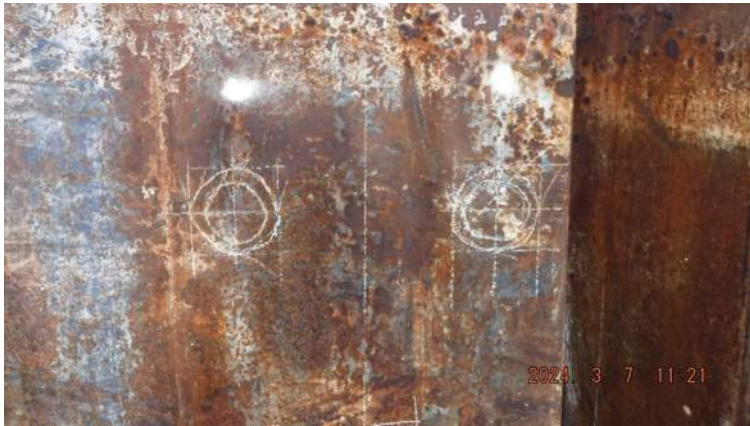
Pier 43: Bridge and Marine crew continued to lay out burn holes for the tie rod and rebar penetrations of P21 of the CWCB
