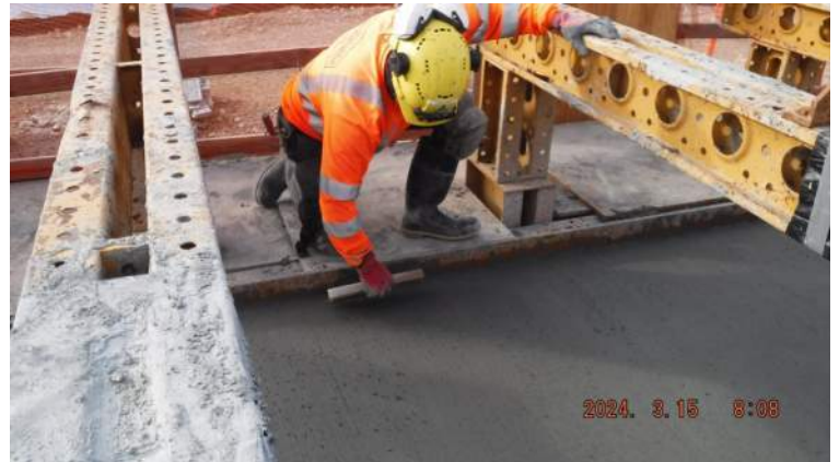
Pier 42: KIWC mason crew used broom for a textured finished of the concrete surface of P14 of the CWCB (STA 8+60 to STA 9+56)
