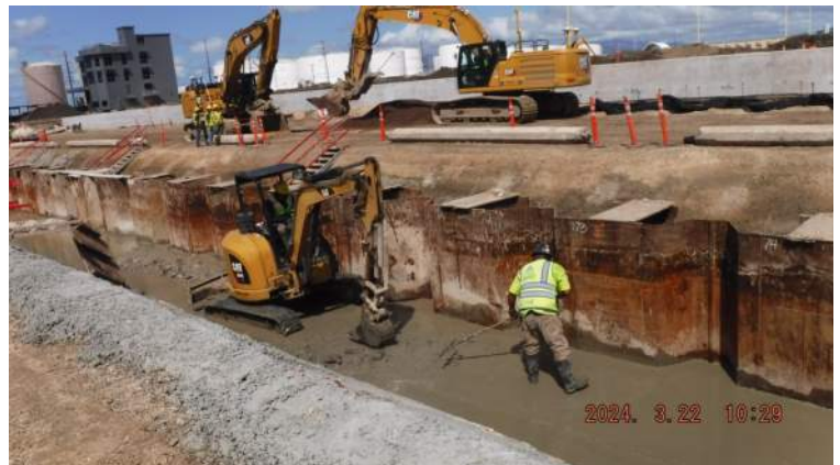
Pier 43: KIWC civil crew removed the muck from P17 to P22 on the ocean side of the combi wall
