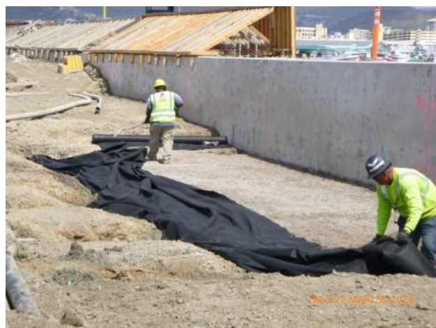
KIWC placing a new section of filter fabric over the cleaned 3b.
