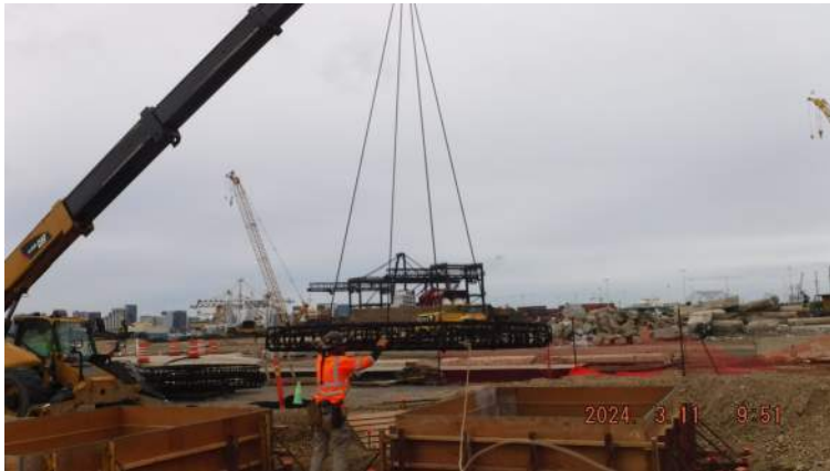
Pier 43: HRSPI crew on site to install the rebar cage for the water line top cover of WL 1 and 2
