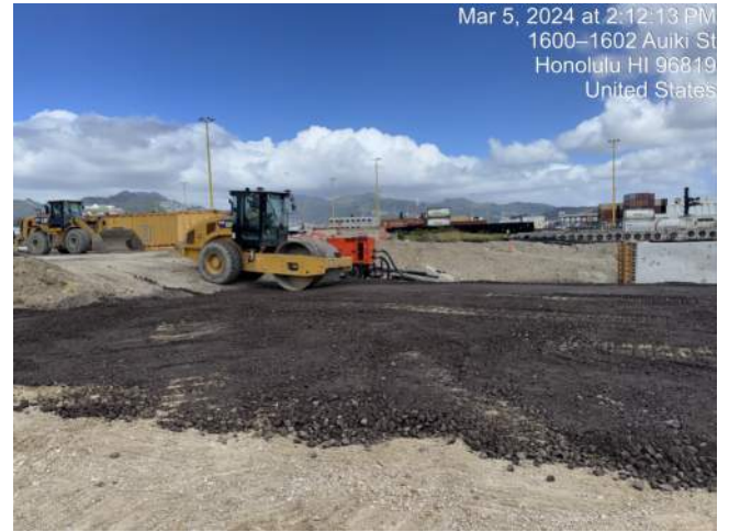
Mar 5, 2024 at 2:12:13 PM 1600-1602 Auiki St Honolulu HI 96819 United States KIWC compacting lift 9 of P0 of the deadman with method compaction
