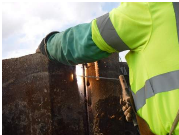
Pier 43: KIWC welder continued to weld th #8 "U" rebar between the sheet pile interlocks
