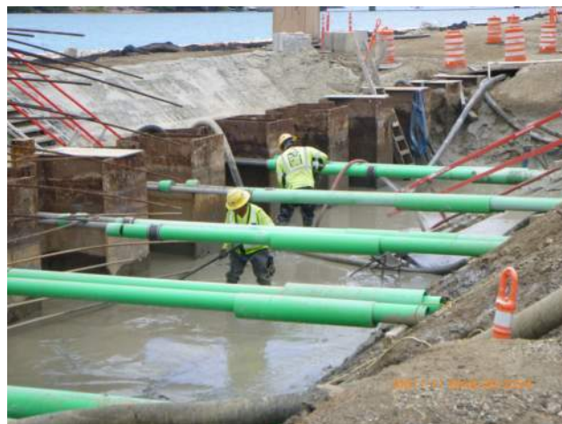
KIWC removing dredge runoff from the landside of the capping beam on pier 42.
