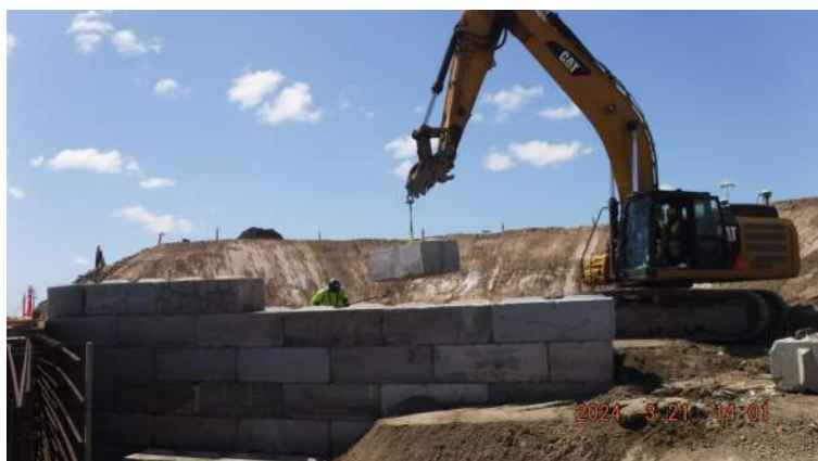
Snug Harbor: KIWC civil crew placed the 6th eco- block for the MSE constructions
