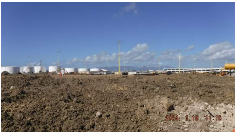
Snug Harbor: Grids 58, 59 and 60 were uncompacted for lift 4 and need to be tested before placing any fill
