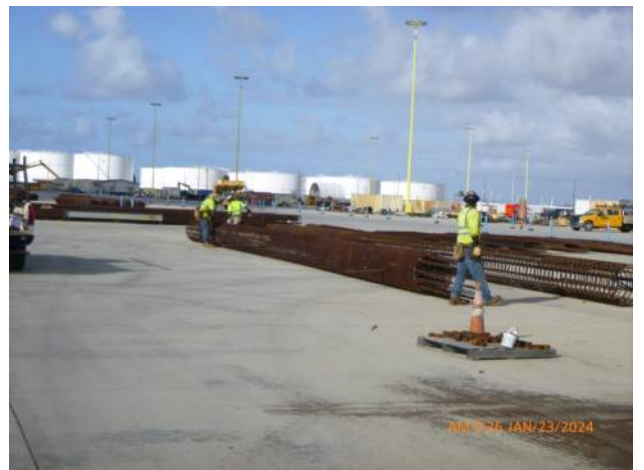
HRSPI installing CSL tubes into the 36" CIDH rebar cages.
