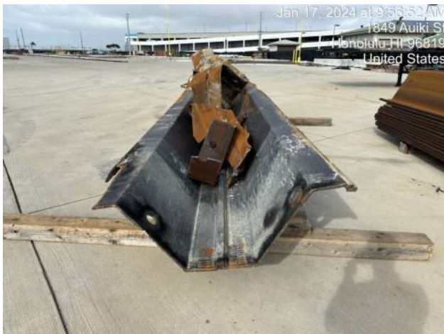
Documentation of damaged sheet pile pulled from Pier 43 location S-74
