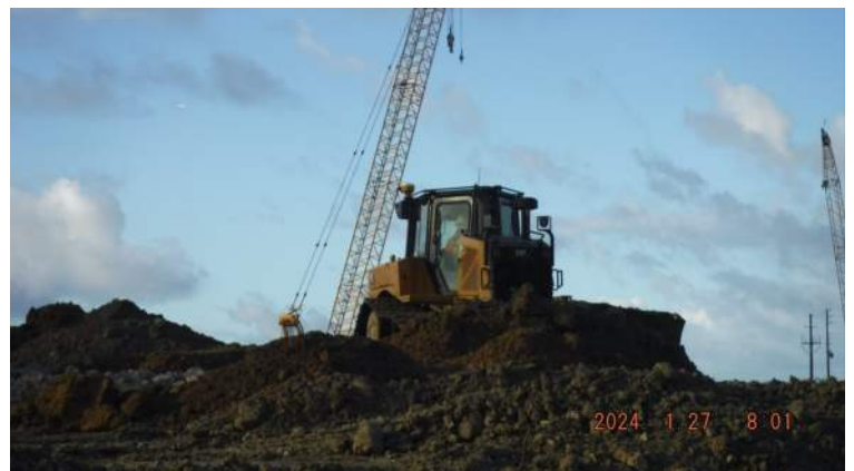
Snug Harbor: The CAT D6 dozer was used to spread the dredged material in 12-inch thick loose lifts
