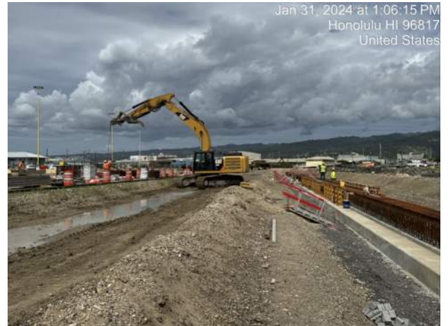
KIWC continued installation of formwork and grates for TD-3 Sta. 3+00 to 4+00
