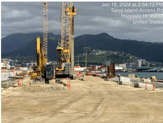
KIWC finished probing using the 63' double king pile
