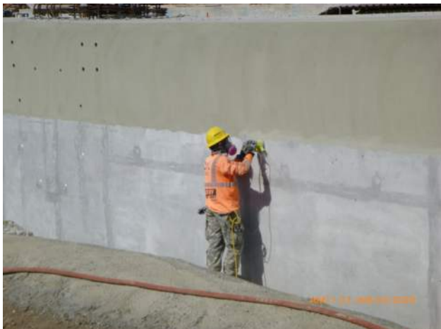
KIWC dry finishing the surface of capping beam pours #6 and 7.
