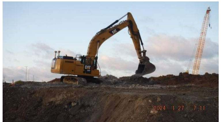
Snug Harbor: KIWC used the CAT 336F excavator's bucket to break down the coral boulders in small pieces
