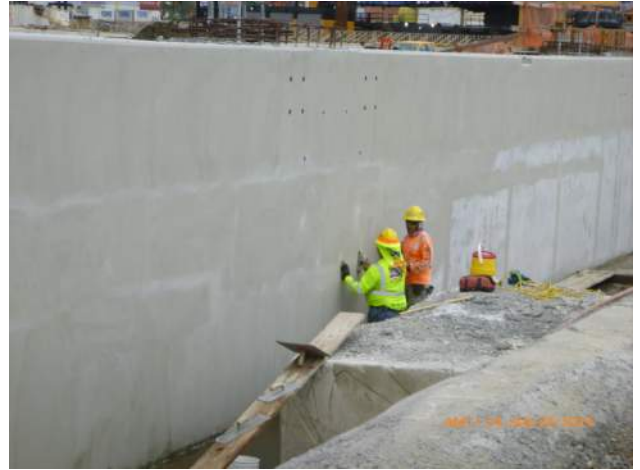
KIWC dry finishing the surface of the capping beam.
