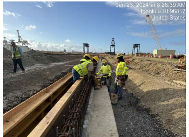
KIWC continued installation of TD-3 formwork from Sta. 3+00 to 5+00
