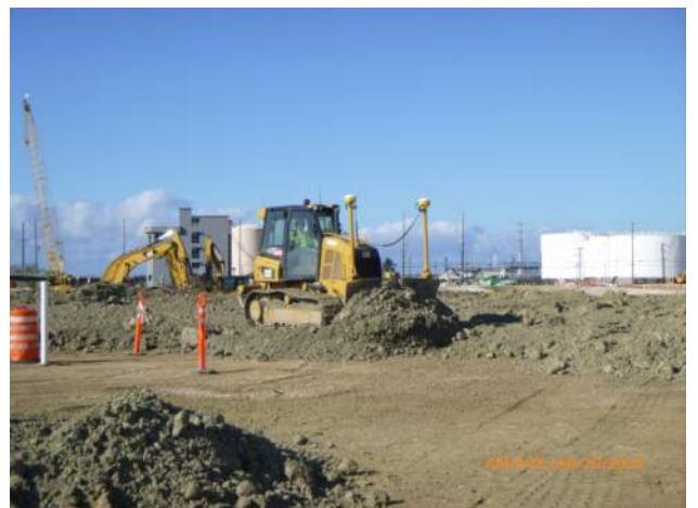
KIWC leveling the surcharge with a track dozer.
