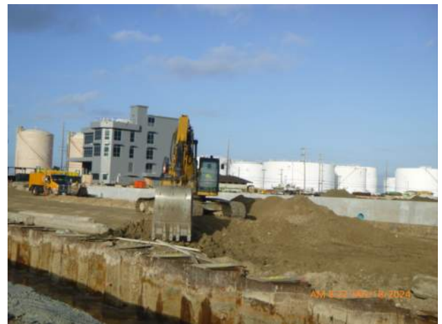
KIWC excavating native material on pier 43.
