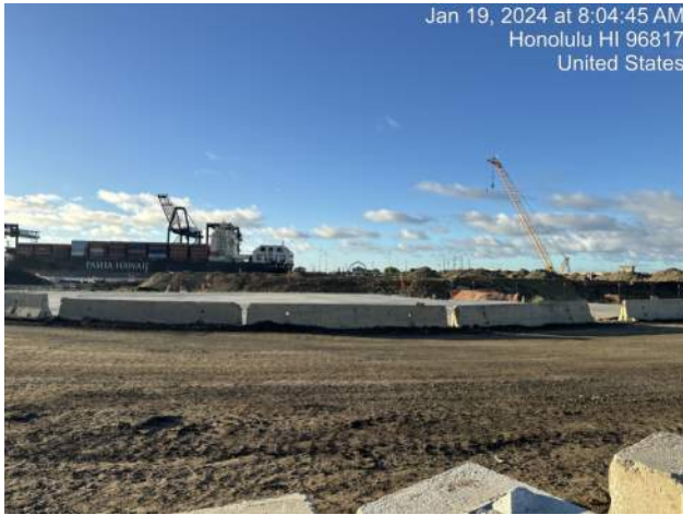
View of Snug Harbor surcharge area
