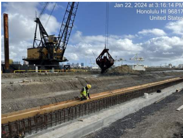
KIWC continued in-water dredging on Pier 41
