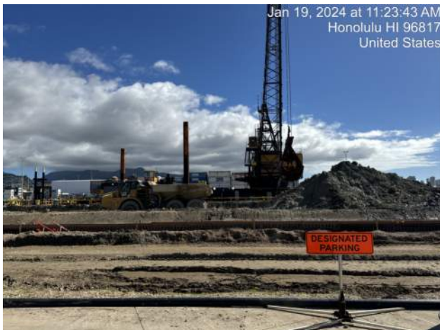
KIWC continued in-water dredging and moving dredge spoils on Pier 41
