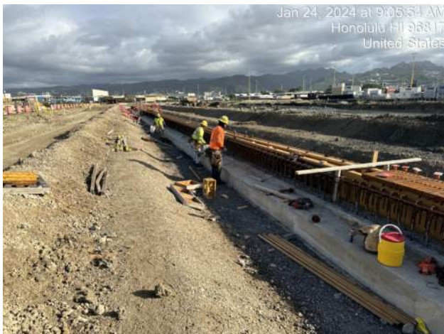
KIWC installing the formwork for TD-3 P3T Sta. 3+00 to 4+00 on Pier 41
