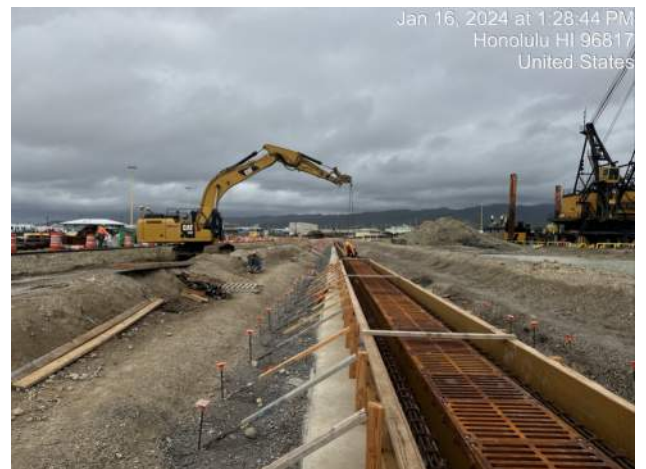
KIWC installing grates for TD-3 P2T Sta. 2+00 to 3+00
