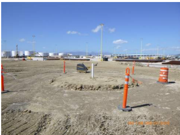
View of compacted fill around the settlement monitors.
