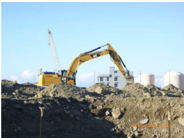
KIWC spreading surcharge with an excavator.
