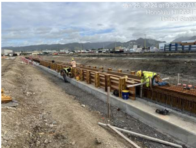
KIWC continued installation of TD-3 P3T on Pier 41
