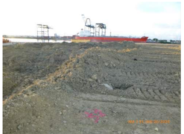
View of surcharge material on snug harbor.
