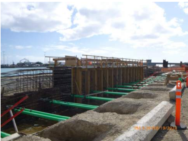
View of formwork around capping beam pour #14.
