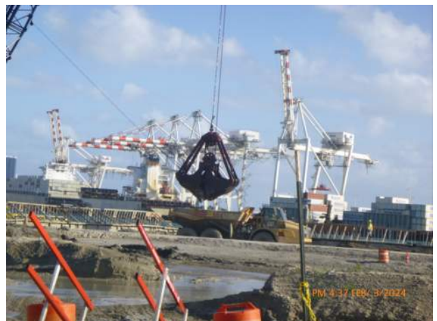
KIWC dredging at the corner of pier 41/42.
