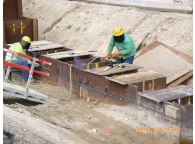
KIWC cutting the continuous king pile wall to top elevation.
