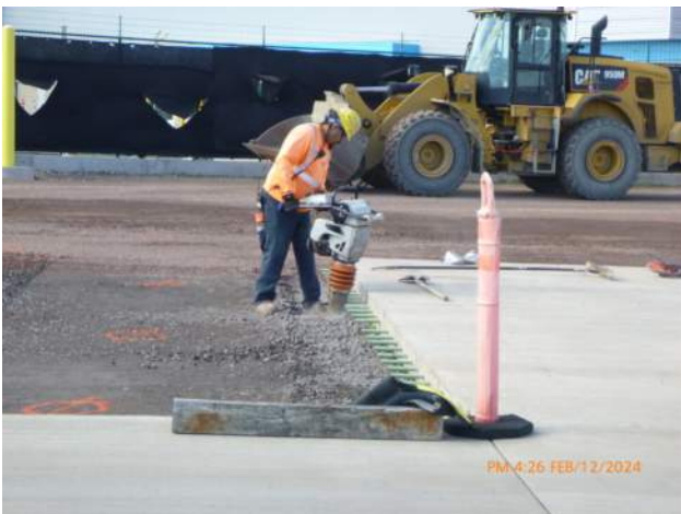
KIWC compacting base coarse around the edge of the blockout.
