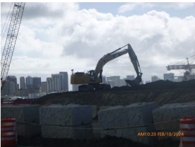
KIWC spreading fill on snug harbor surcharge.
