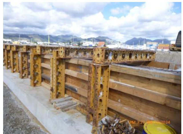
View of formwork installed around TD-3 pour #4 walls.
