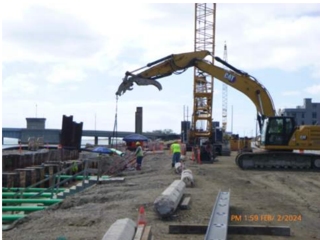
KIWC setting tie rods through the combi wall.
