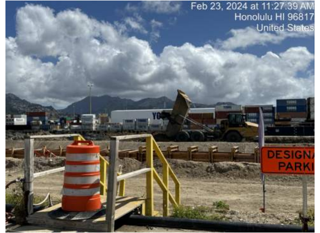
KIWC continued placing dredge spoils on Pier 41
