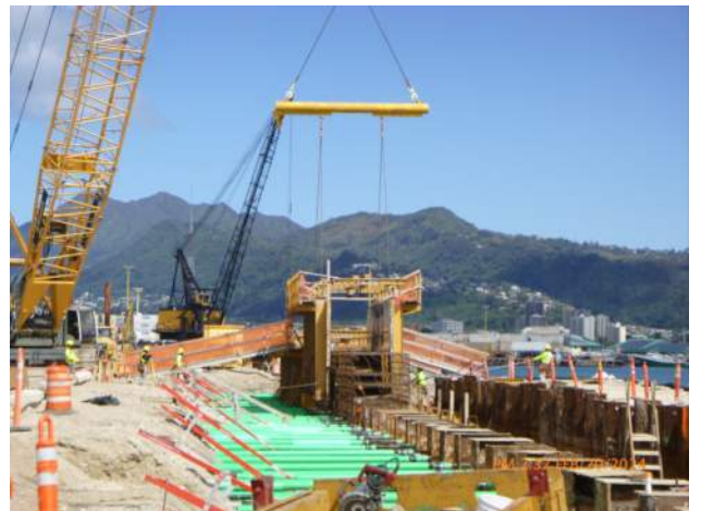
KIWC setting formwork around capping beam pour #14.
