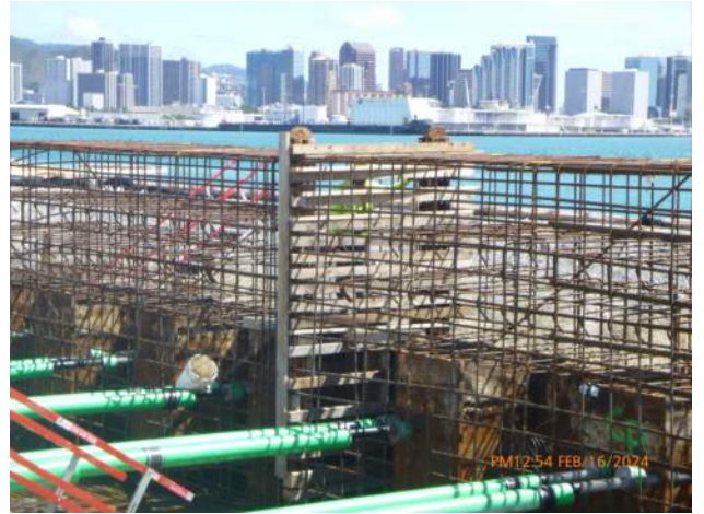
KIWC installing formwork at capping beam pour #14 CJ's.
