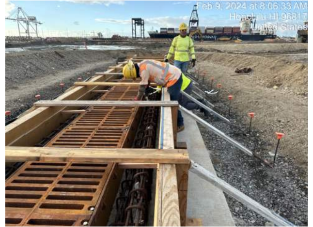
KIWC installing the waterstop for TD-3 P1T Sta. 1+00 to 2+00
