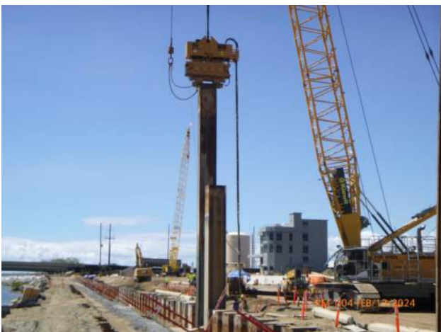
KIWC pulling up KP-065 to check the interlock.
