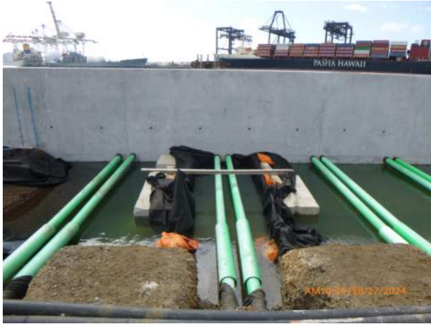
View of formwork for CLSM cutoff wall.
