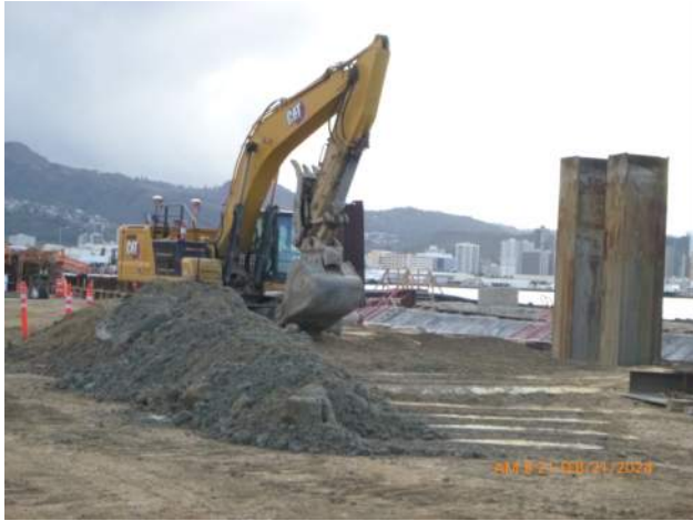
KIWC building a berm around the SP-074 excavation.
