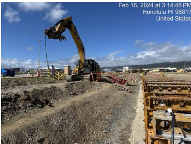
KIWC placing grates and frames for TD-3 P4T on Pier 41
