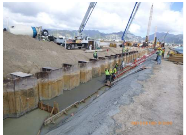
KIWC pouring a mud mat on the waterside of the LSCRB.
