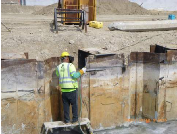
KIWC cutting the top of the combi wall to top elevation.
