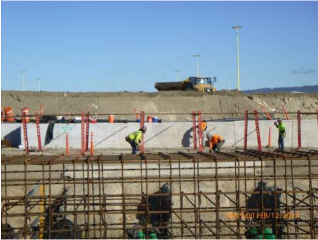
HRSPI fabricating the rebar cage for the capping beam.
