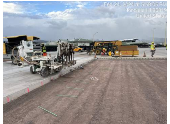
KIWC finished drilling dowels in the "H1" blackout for the shift
