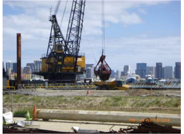
KIWC dredging at the corner of pier 41/42.
