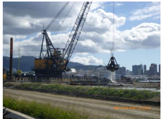
KIWC dredging along pier 41.
