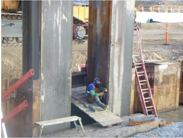
KIWC repairing interlocks on double king pile KP-066.
