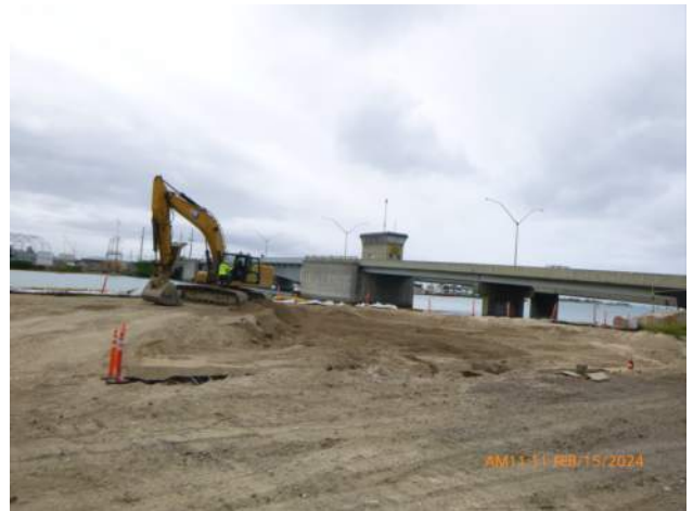
KIWC excavating the stone column work pad on pier 43,
