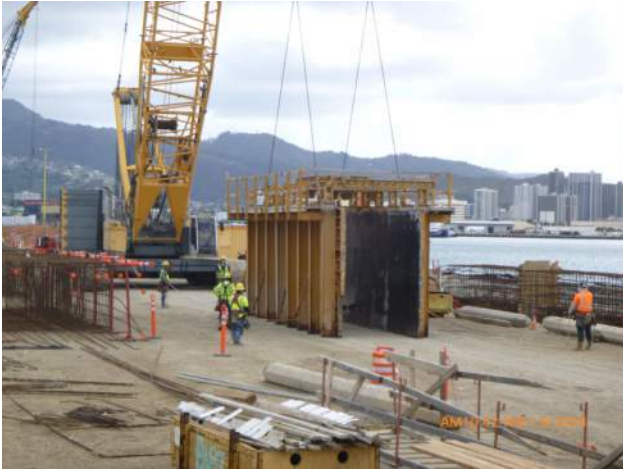
KIWC staging formwork for capping beam pour #14 on pier 42.
