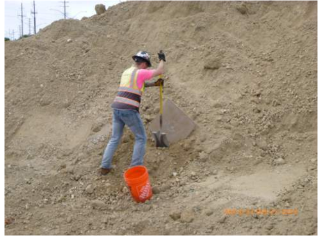
MPE taking a soil sample on pier 43.
