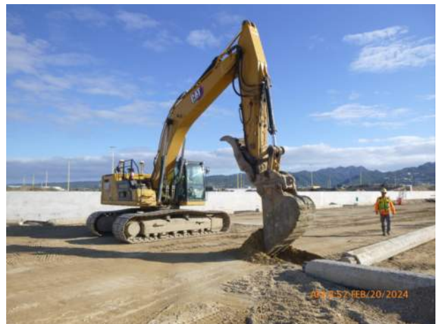
KIWC trenching for tie rods on pier 43.
