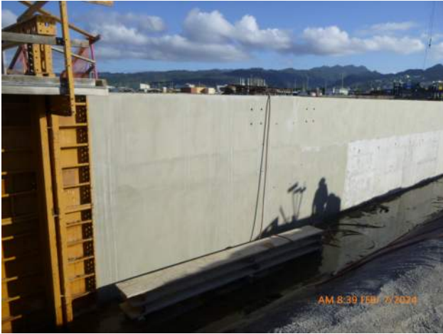
View of dry finish on capping beam pour #5.
