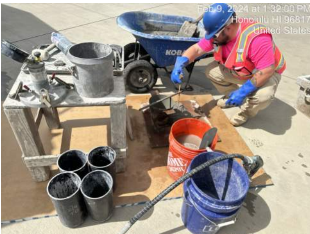
MPE performing concrete testing for the TD-3 pours
