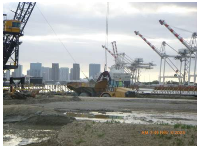
KIWC dredging at the corner of pier 41/42.
