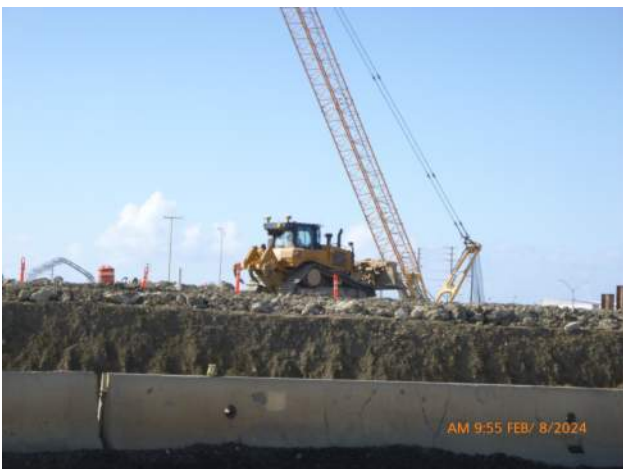
KIWC grading and leveling the 6th lift of backfill.
