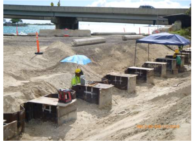
KIWC cutting the combi wall to top elevation.
