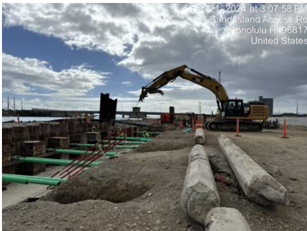
KIWC continued installation of tie rods on Pier 43
