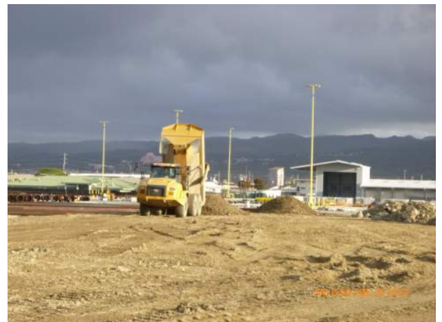
KIWC placing the 6th lift of surcharge over snug harbor.
