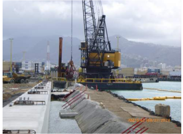
KIWC dredging along pier 42.
