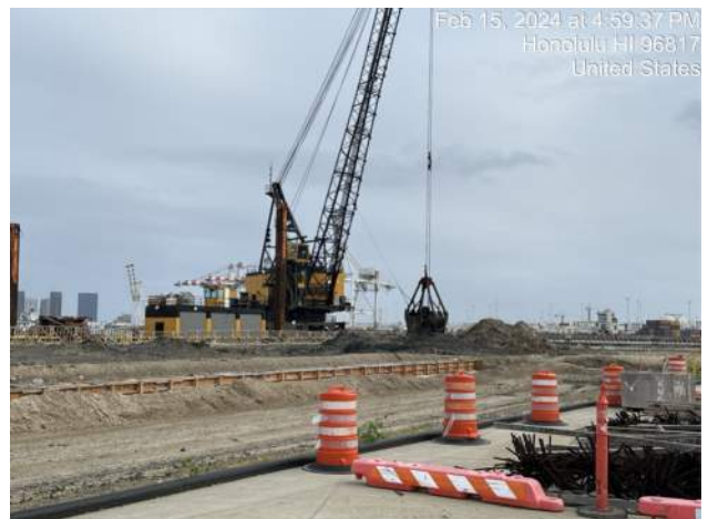
KIWC continued in-water dredging on Pier 41
