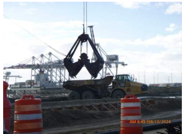
KIWC dredging along pier 41.
