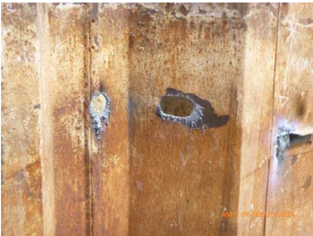
KIWC burning tie rod penetrations through the combi wall on pier 43.
