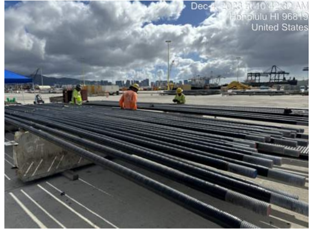
KIWC repairing the tie rod tape wrap on the PCC
