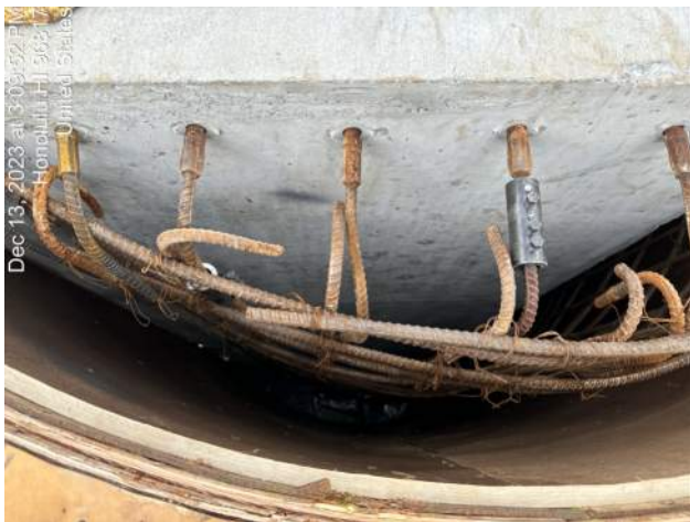
KIWC progress installing rebar couplers for the P42 corner reinforcement
