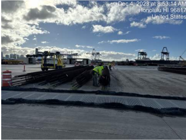
HRSPI installing CSL tubes for the 36" rebar cages on the PCC
