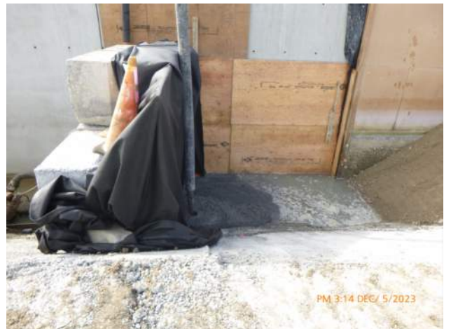
KIWC pouring a cutoff wall near the corner of pier 41/42.
