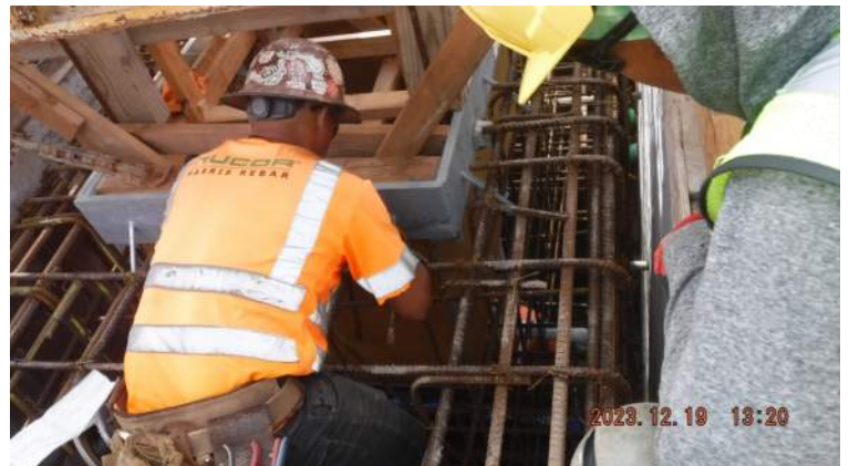
2023.12.19 13:20 Pier 42: HRSPI reinstalled the rebars for the utility vault in P5
