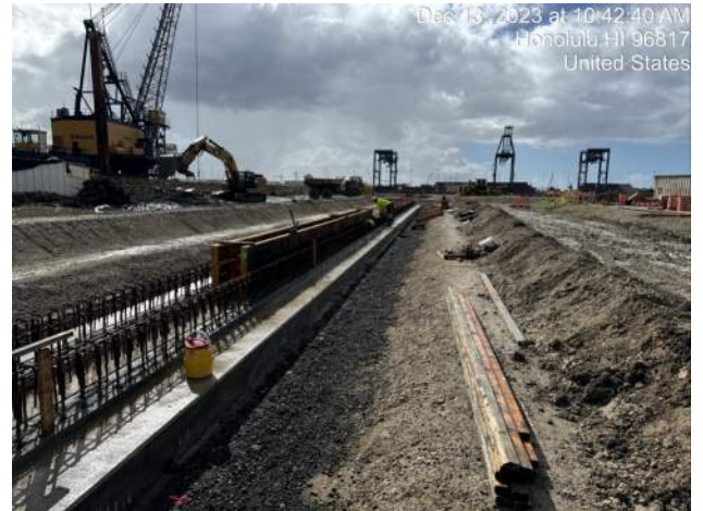
KIWC progress installing formwork for P2T of TD-3 on Pier 41
