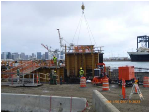
KIWC installing formwork around capping beam pour #11.
