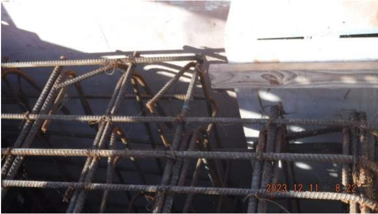
Pier 42: P-11 KIWC carpentry crew installed bulk head and expansion sheet
