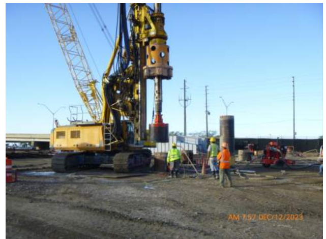
KIWC cleaning out the bottom of CIDH shaft 14-A1-48A.
