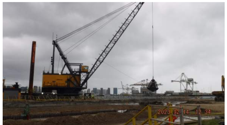
Pier 41: DB Seattle continued in water dredging at approximately STA 18+00 to 19+50
