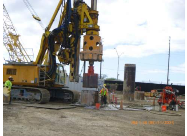
KIWC cleaning out the bottom of cage 14-A1-48A.
