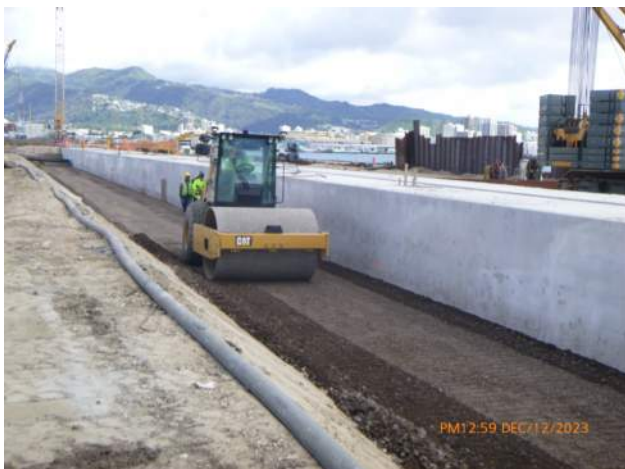
KIWC backfilling and compacting on the landside of the P43 LSCR.
