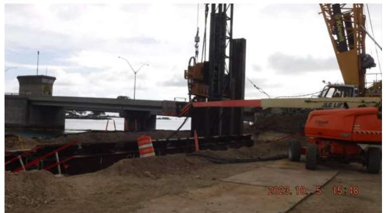
Pier 43: KIWC Bridge and Marine crew stopped pile driving for today
