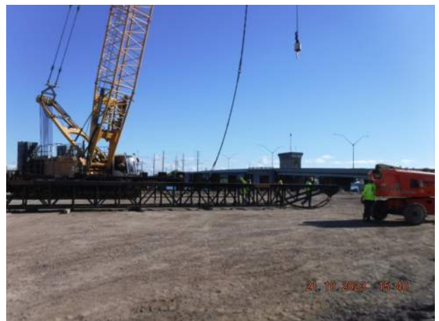
KIWC finished driving all sheet piles on the CWCB
