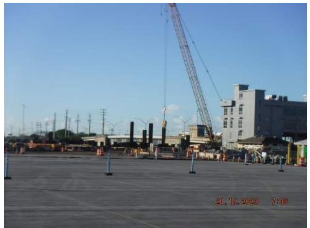
KIWC driving sheet piles for the CWCB on Pier 43
