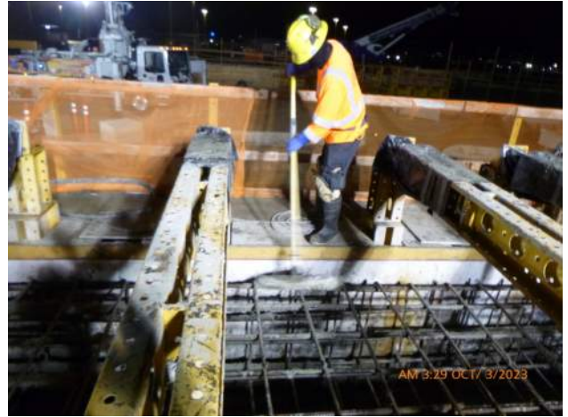
KIWC striking off excess concrete from the top mat.
