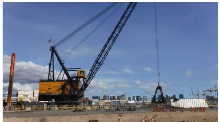
Pier 41: KIWC DB Seattle continued in water dredging
