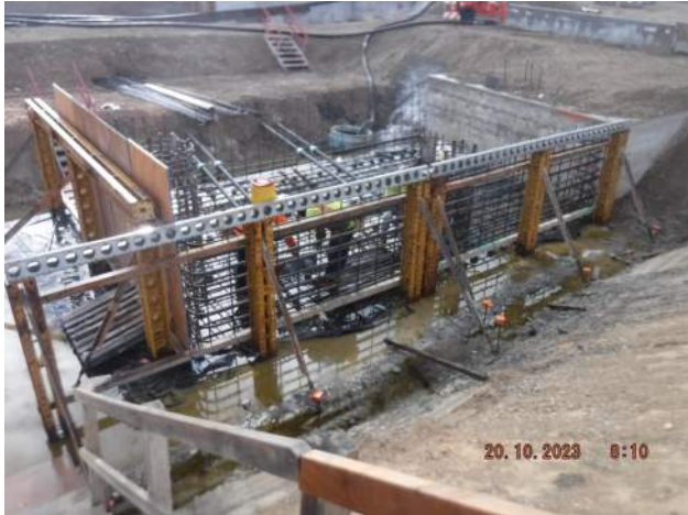
HRSPI installing the grillage for P0 of the deadman on Pier 41
