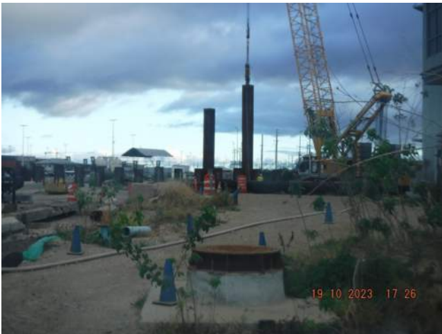
KIWC driving sheet piles using the APE vibratory hammer on Pier 43
