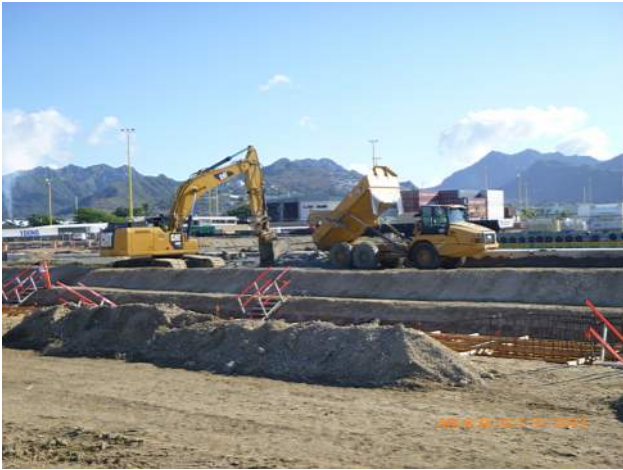
KIWC stockpiling dredged material on pier 41.
