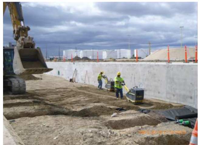
KIWC backfilling over tie rods in snug harbor.
