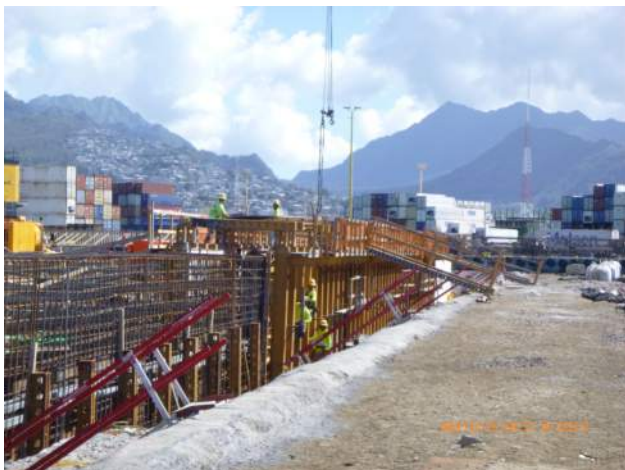
KIWC loosening formwork around Pier 42 capping beam pour #4.
