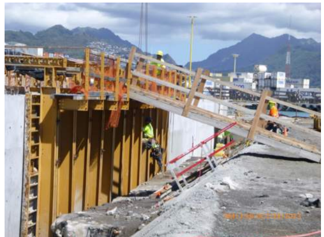
KIWC removing formwork from around capping beam pour #3.
