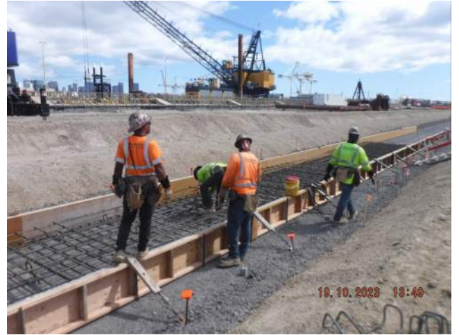
HRSPI installing reinforcement for the trench drain from Sta. 6+00 to 3+40
