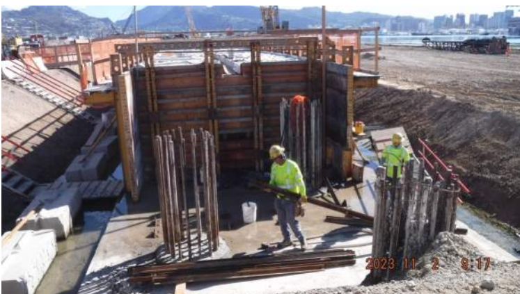
Pier 43: KIWC carpentry crew continued pre stripping Pour #6 of the LSCRB
