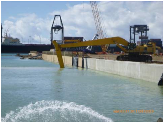
KIWC dredging along the pier 41 capping beam.
