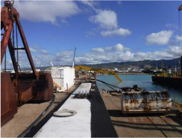
KIWC performing landside dredging on Pier 41
