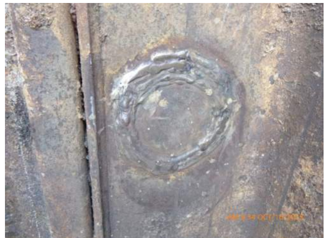
View of fillet weld repair on 4.5" diameter penetration through combi wall.
