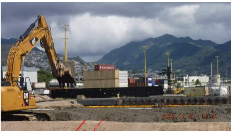
Pier 41: Dredged material was dumped on the wst side of the K-rail
