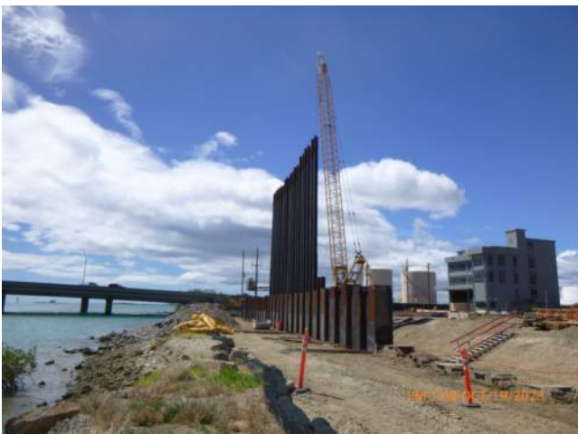
KIWC threading sheet piles along the combi wall alignment on pier 43.
