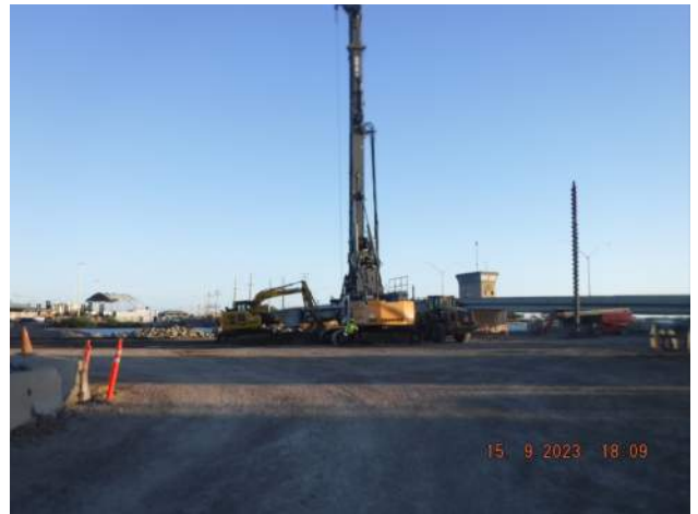
KIWC predrill crew departing from the site
