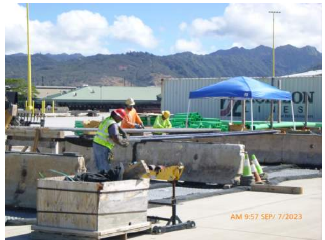
KIWC wrapping tie rods on the PCCP.
