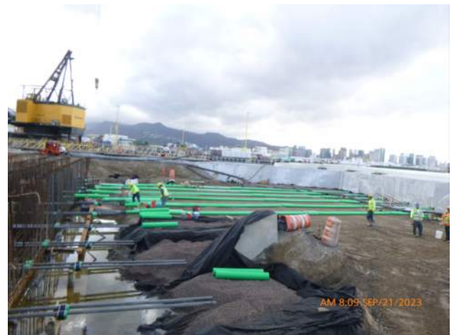
KIWC installing tie rods between LSCRB pour #1 and the capping beam.
