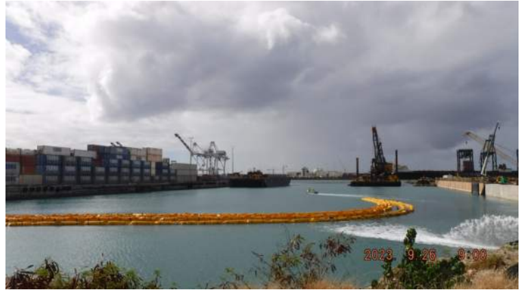
Pier 41: Bridge and Marine crew moved the silt curtain storage from the west (Pier 41) to the east (Pier 40)
