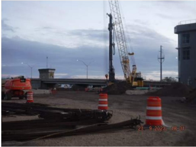
KIWC departed from the site
