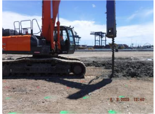
KNA predrilling a pilot hole prior to predrilling to depth
