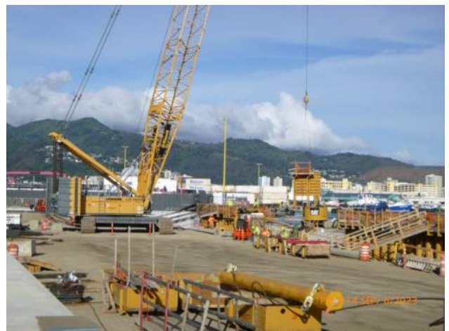
KIWC removing formwork from around P42 capping beam pour #1.
