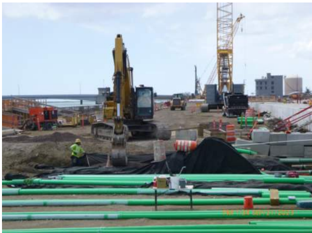
KIWC excavating for tie rods on pier 42.
