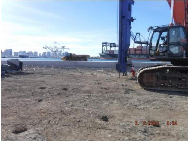
KNA installing wick drains in the Snug Harbor surcharge area
