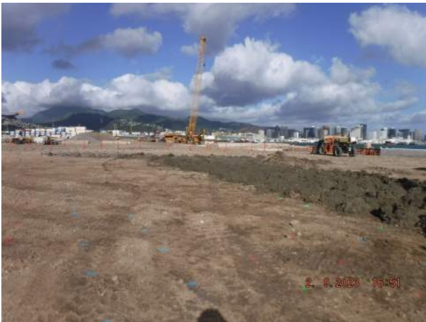
KNA progress predrilling this shift
