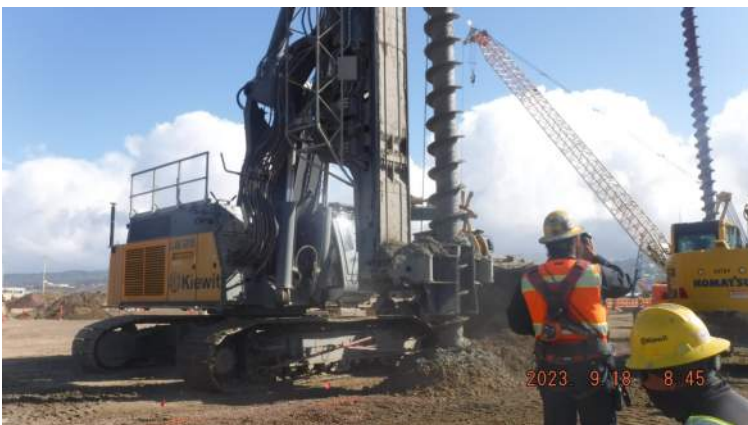
Pier 43: KIWC foundation crew continued to predrill the combi wall
