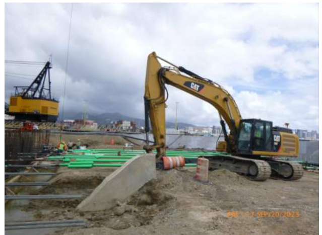
KIWC trenching for tie rods on pier 42.
