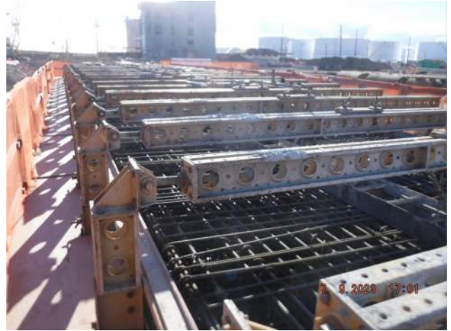
View of the LSCRB rebar and formwork on Pier 43
