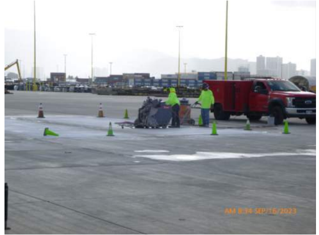
NCS sawcutting PCCP blockouts on the pavement.
