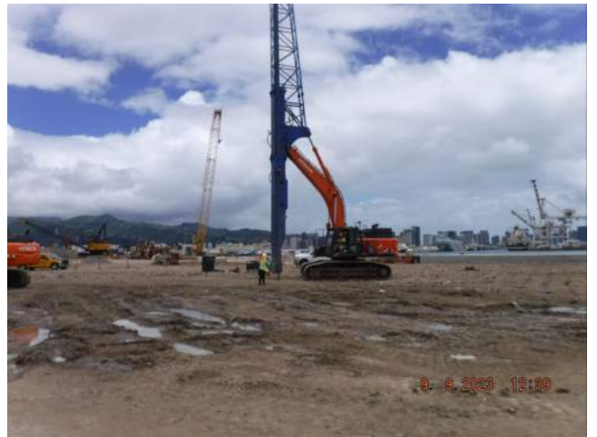
KNA installing wick drains 47' bgs in the Snug Harbor surcharge area
