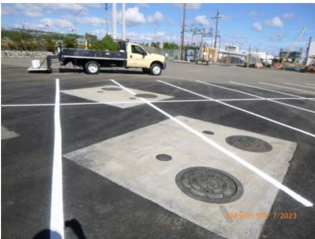
APL striping the P51 parking lot.
