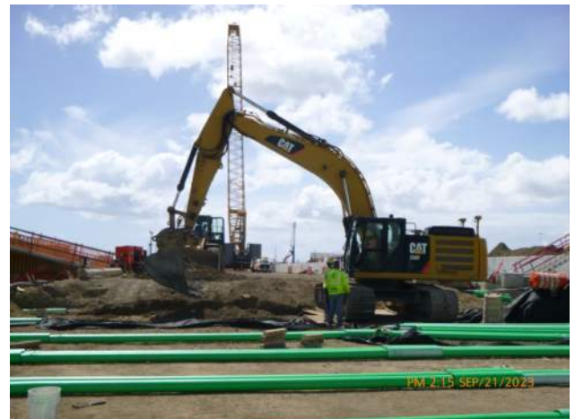
KIWC excavating for tie rods on pier 42.
