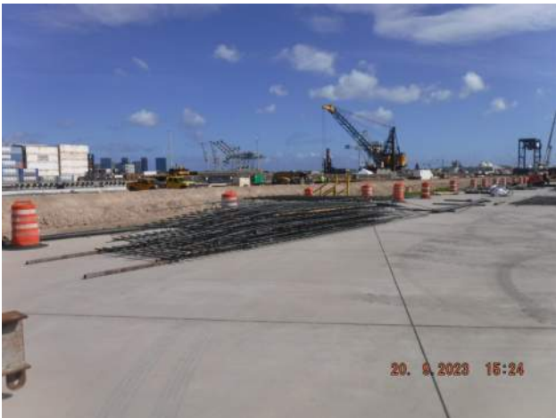
HRSPI progress fabricating rebar cages for the trench drain on Pier 41
