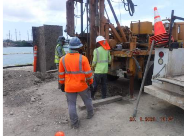
KG drilling location 173 for SPT testing on Pier 43
