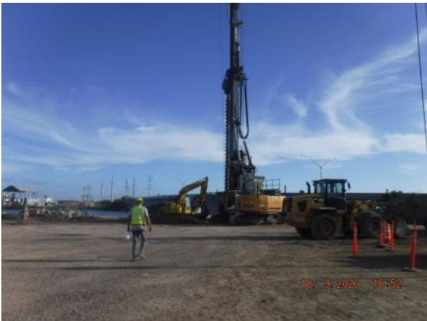
KIWC predrilling for installation of the combi wall piles on Pier 43
