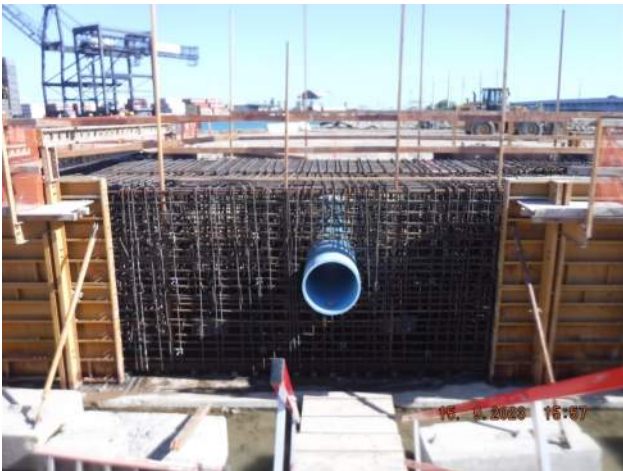
View of the utility blockout in the LSCRB P6 on Pier 43
