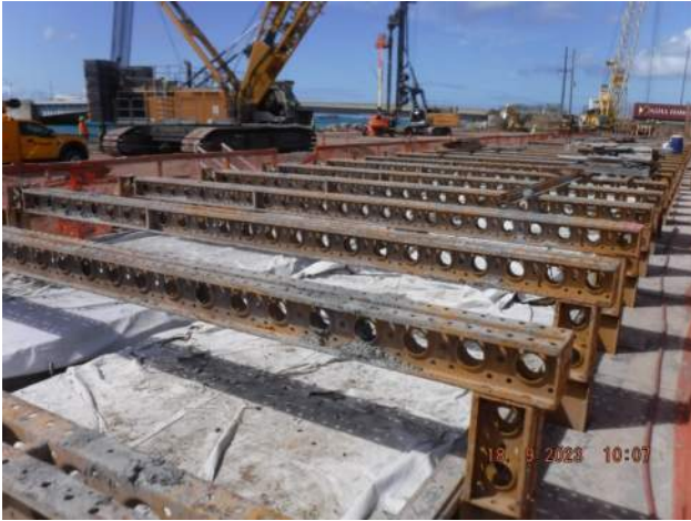
View of the LSCRB P5 on Pier 43
