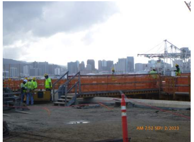
KIWC installing formwork around the pier 43 LSCRB pour #5
