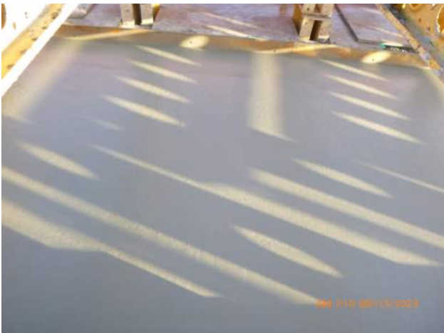
KIWC finishing the surface of capping beam pour #4 on pier 42.
