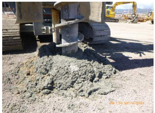
KIWC predrilling for the combi wall on Pier 43.
