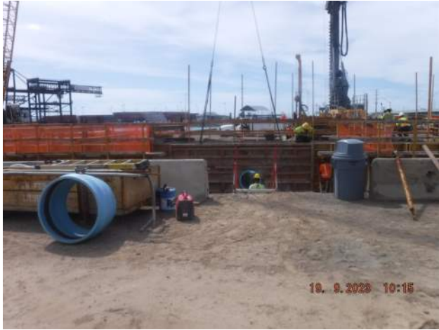
KIWC continued installation of the LSCRB P6 on Pier 43
