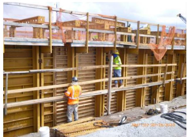
KIWC installing formwork around capping beam pour #3.
