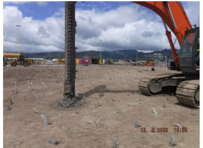
KNA predrilling remediation locations for the wick drain installation
