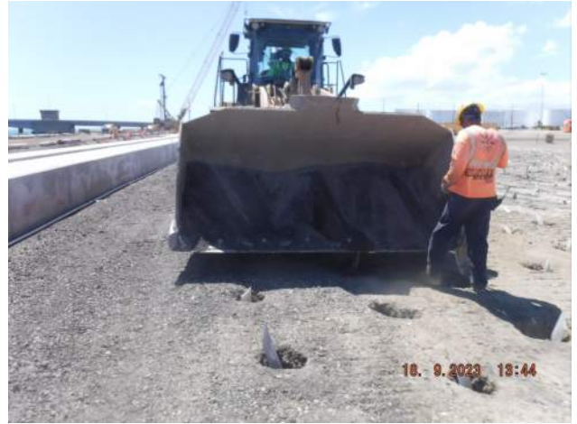
KIWC backfilling wick drains in the Snug Harbor surcharge area
