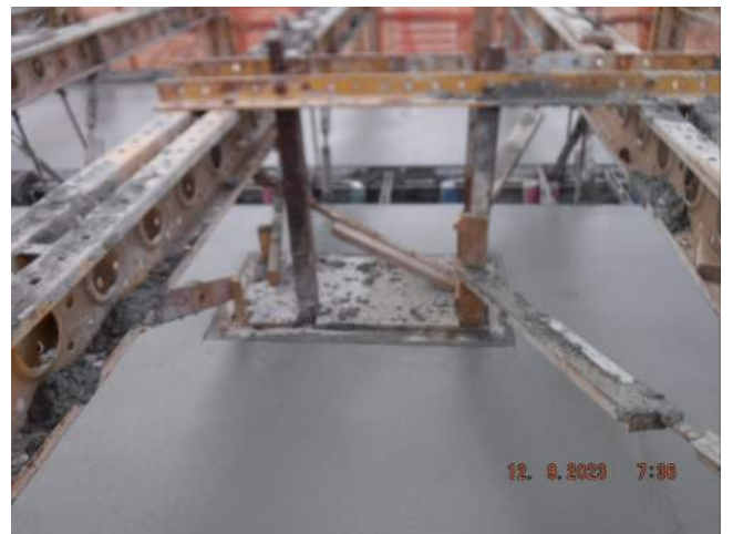
View of P5 of the LSCRB on Pier 43
