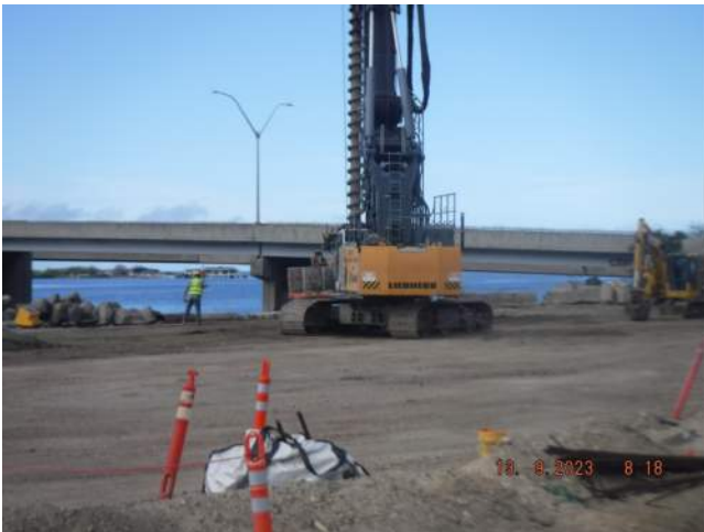
KIWC continued predrilling for installation of the combi wall on Pier 43
