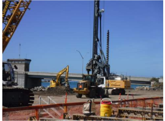
KIWC predrilling for installation of the combi wall on Pier 43
