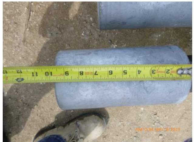
View of tie rod coupler.
