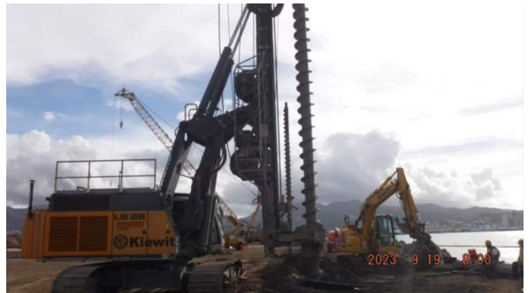
Pier 43: KIWC Foundation crew continued to predrill for the combi wall
