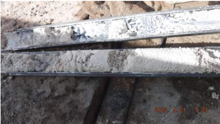
Pier 43: Recovered sample from the SPT sampling consisted of white coralline silty sand and gravel from 30.5'bgs
