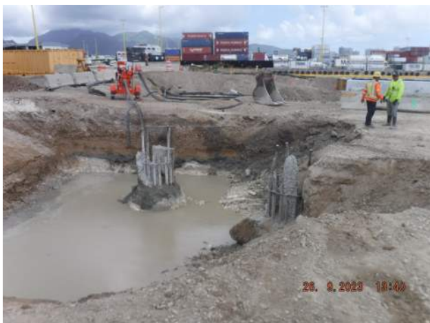
KIWC progress excavating P0 of the deadman on Pier 41
