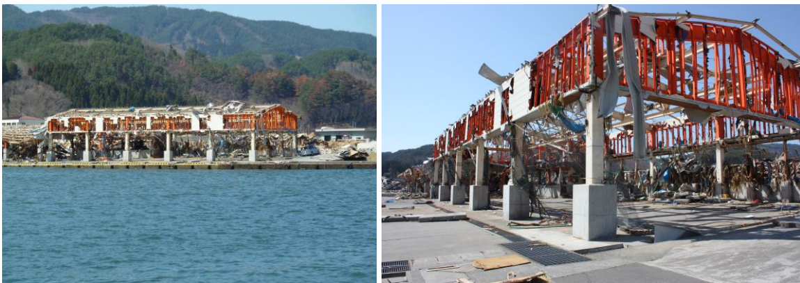
Figure 2-36: Cladding stripped from steel-framed warehouse in Taro Harbor.
