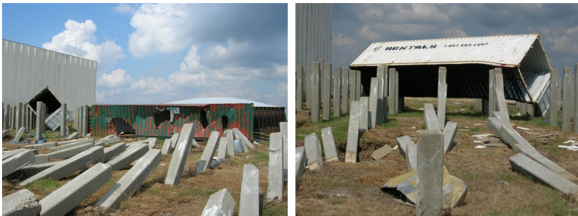
Figure 2-13: Damage to precast piles due to impact and damming effects of floating shipping containers in Biloxi, Mississippi
