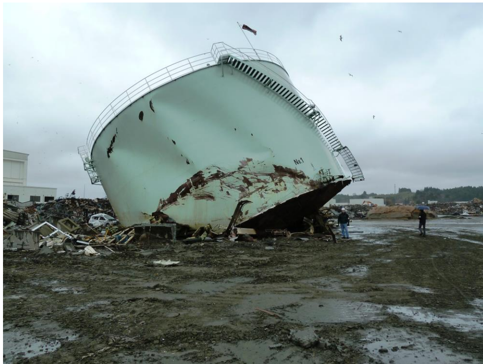
Figure 2-30: One of many large fuel storage tanks in Kesennuma Harbor damaged during the Tohoku Tsunami
