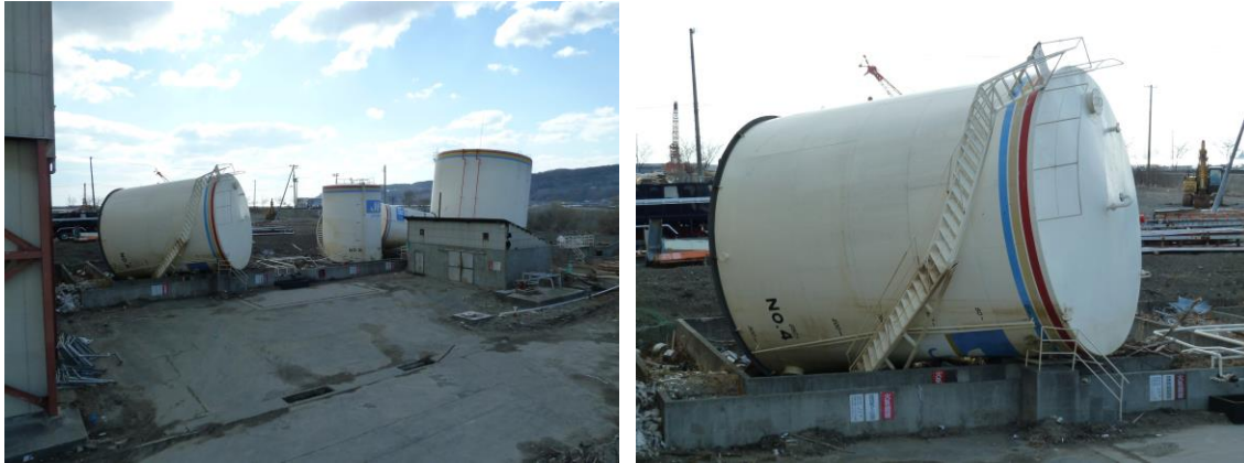
Figure 2-29: Damage to fuel storage tanks at Kuji Port during the Tohoku Tsunami
