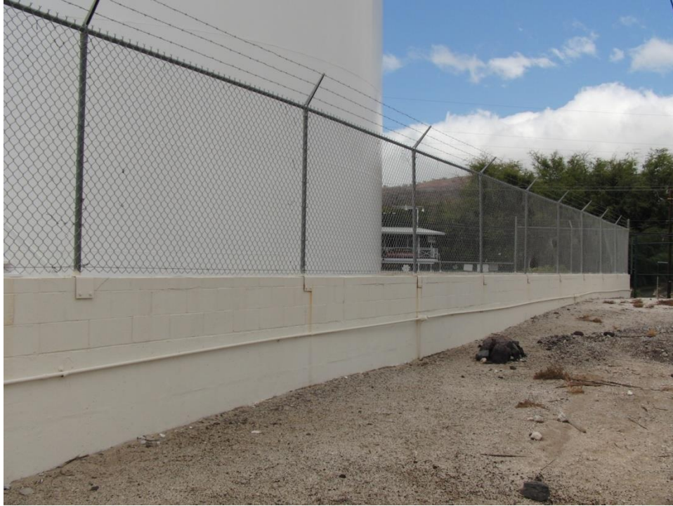
Figure 4-112: CMU wall surrounding Midpac fuel storage facility
