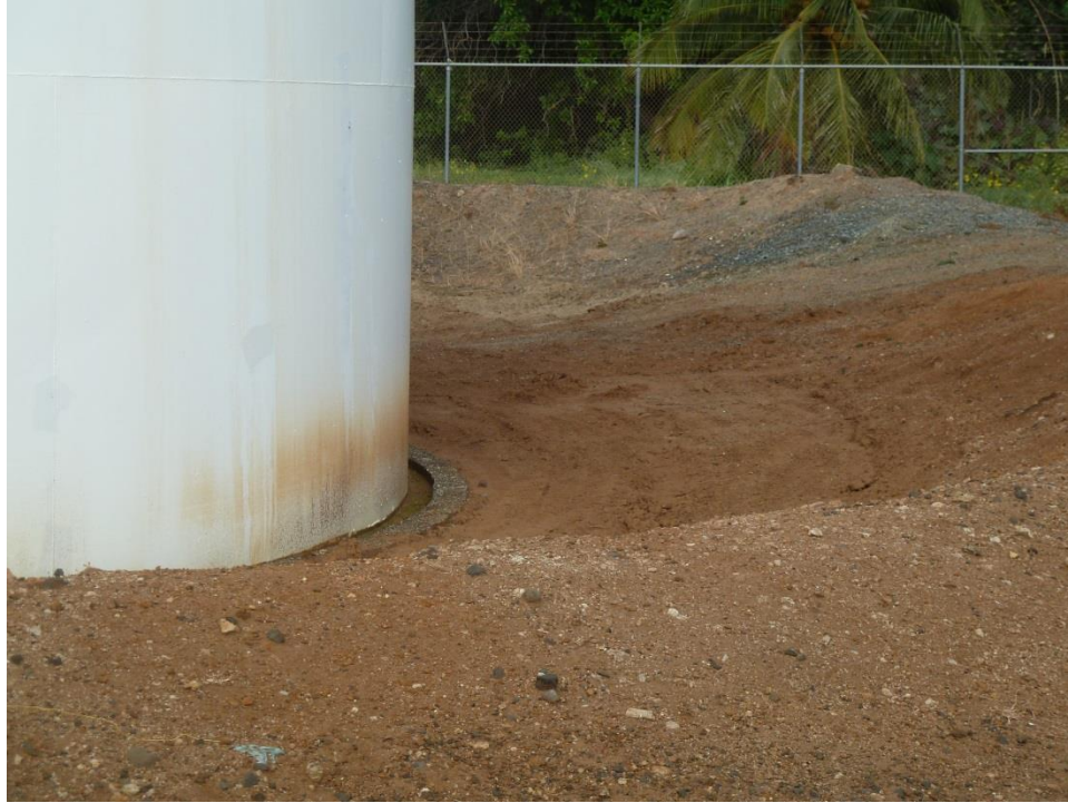
Figure 4-11: Midpac fuel storage tank base and containment berm
