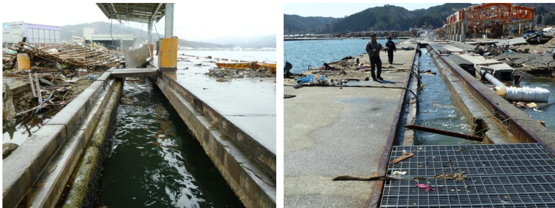
Figure 2-25: Concrete and steel grating “breakaway” panels uplifted by the Tohoku Tsunami in Kesennuma harbor (left) and Taro harbor (right)
