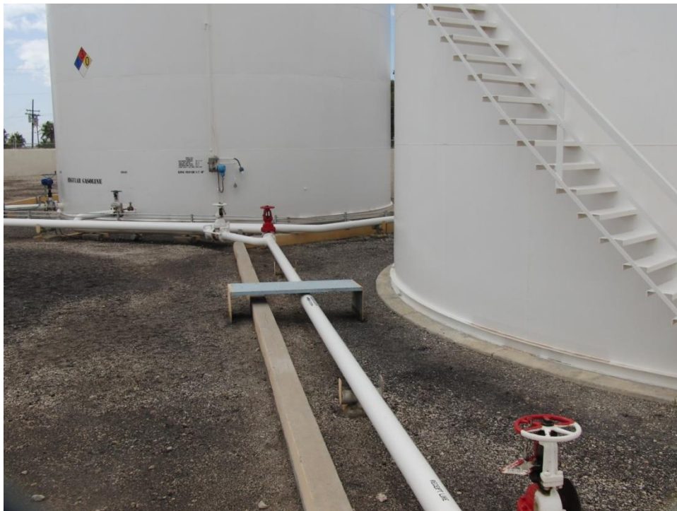
Figure 4-113: Base support and piping in Midpac tank farm
