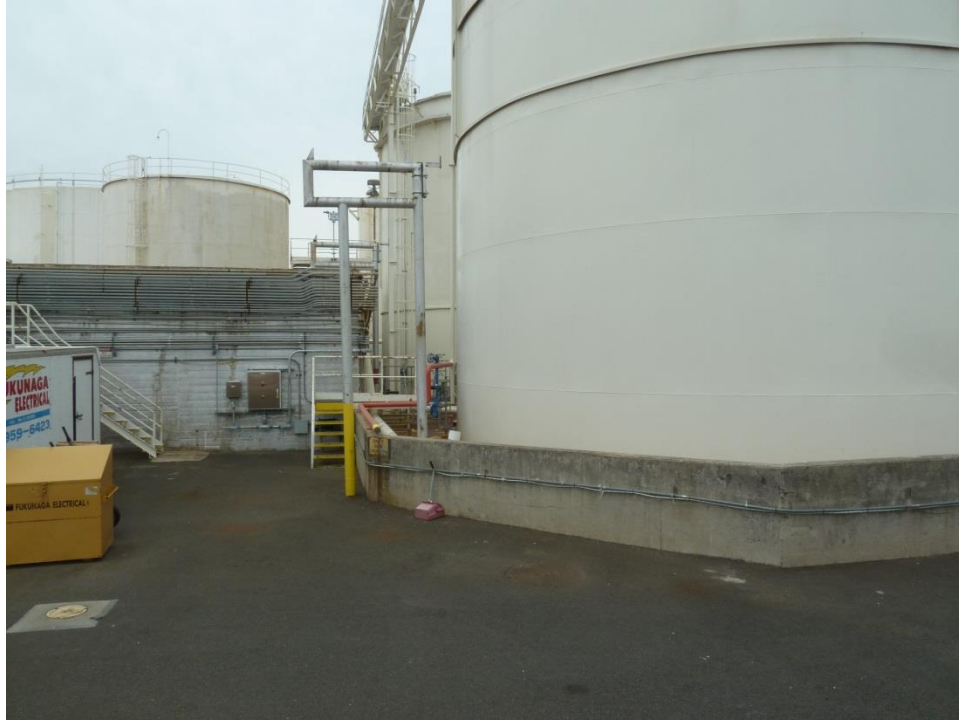
Figure 4-49: Chevron ship fuel storage tanks with 3 ft. and 10 ft. high containment walls
