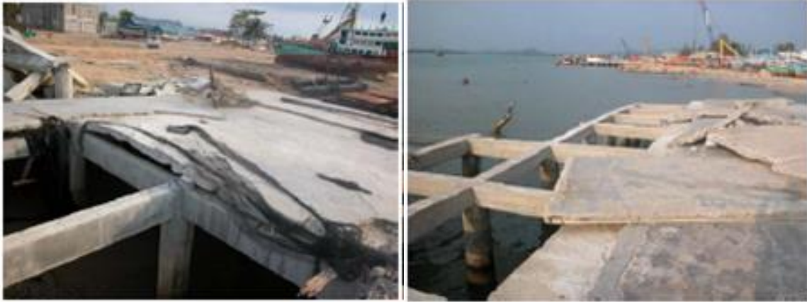
Figure 2-24: Tsunami uplift damage to precast harbor piers in Kao Lak, Thailand
