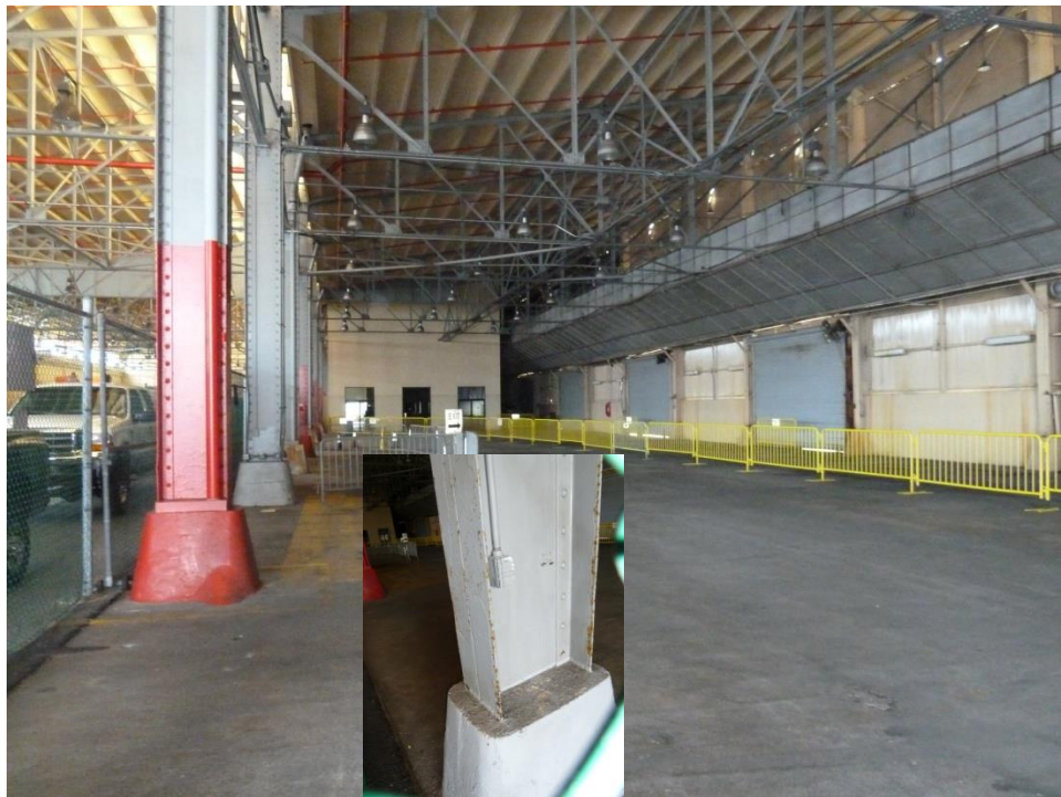
Figure 4-89: Interior of Pier 1 Warehouse and typical column base (inset)
