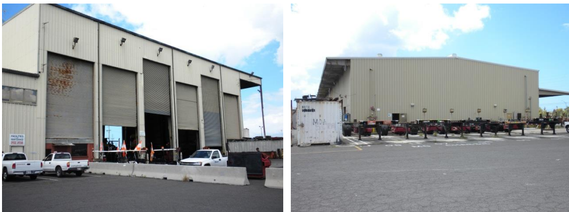
Figure 4-62: Pre-manufactured steel framed warehouses on Sand Island
