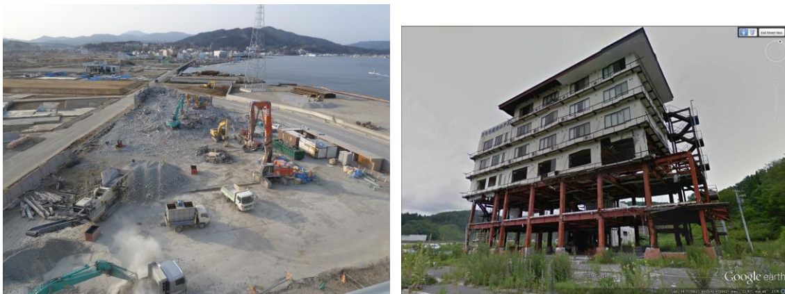
Figure 2-40: Demolition of Kesennuma vertical evacuation building in March 2013 (left) and unrepaired state of Taro Hotel from Google Earth street view July 2013 image (right).
