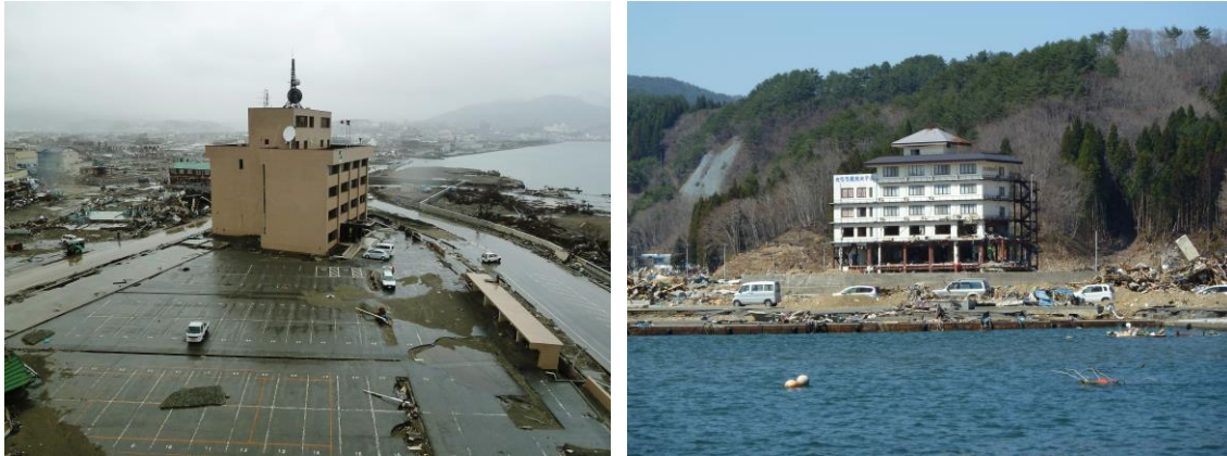
Figure 2-39: Multi-story buildings that survived inundation to the third floor level; Reinforced concrete vertical evacuation building in Kesennuma Harbor (left) and steel-framed hotel adjacent to Taro Harbor (right).
