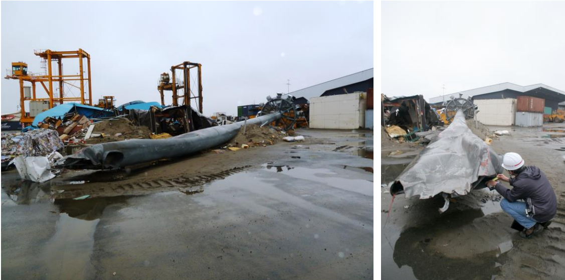
Figure 2-18: Impact damage to large light standard in the Sendai Harbor shipping container yard.
