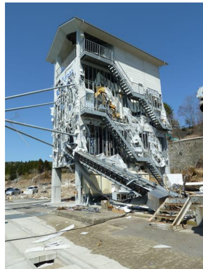
Figure 2-38: Port buildings with intact structural elements but extensive cladding damage; Kesennuma (left) and Taro (right)
