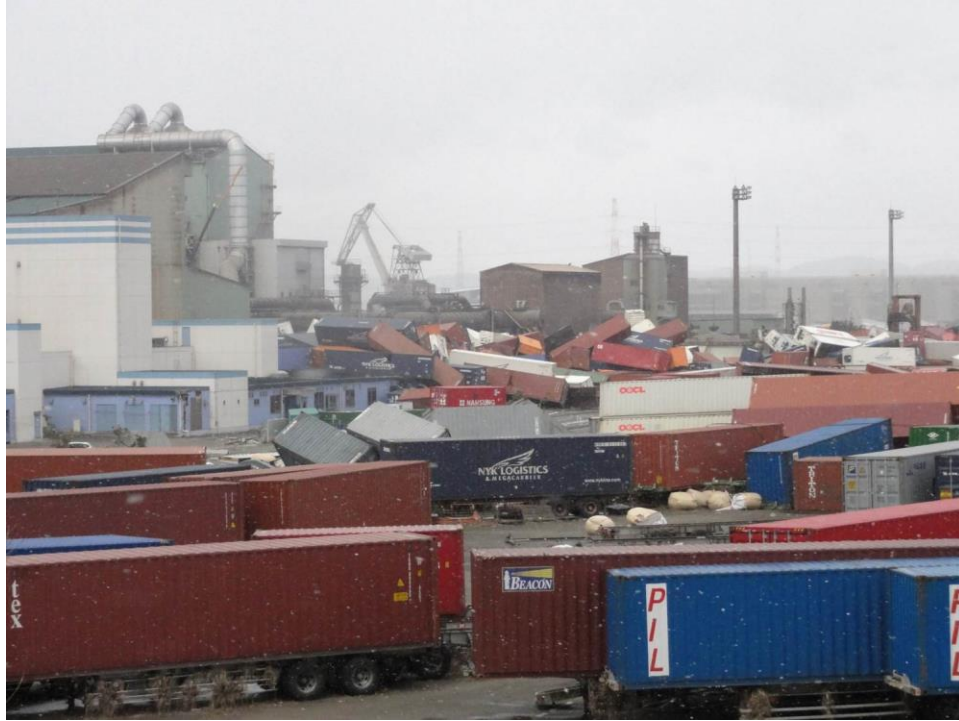
Figure 2-16: Shipping containers impacting port buildings in the Sendai Harbor after the Tohoku Tsunami
