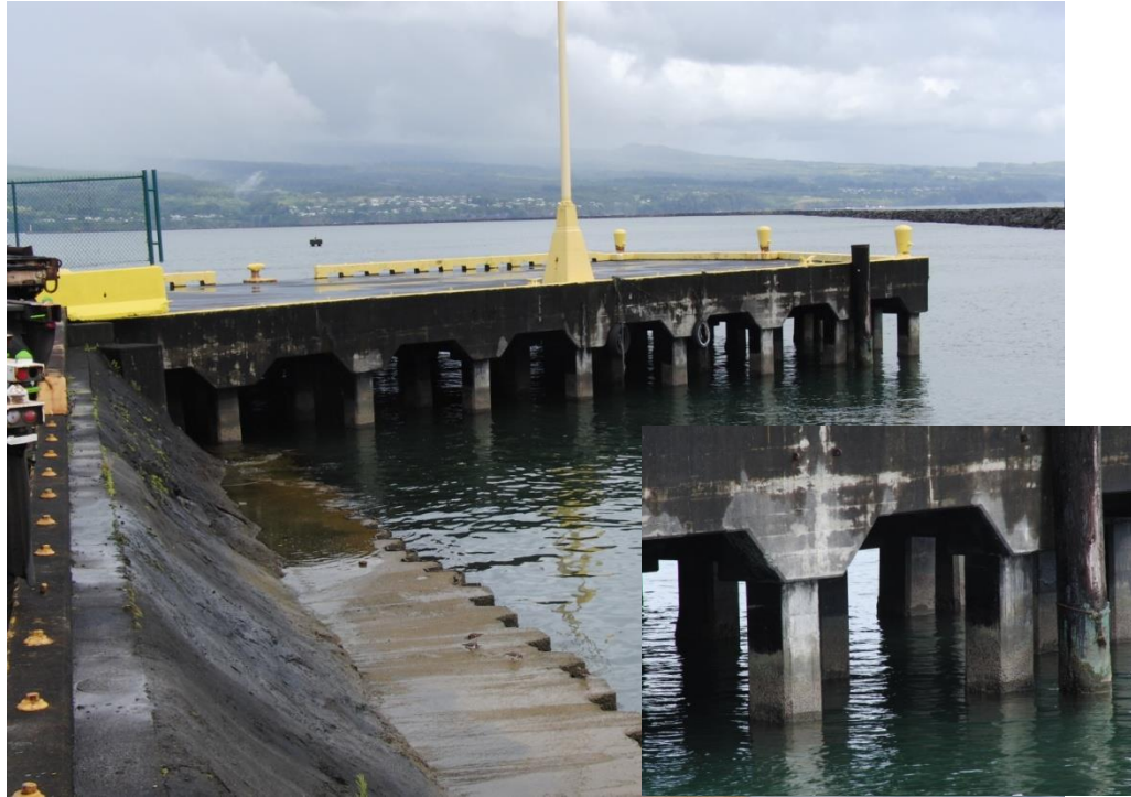
Figure 4-95: Pier 1 newer construction with view of pile to deck connection (inset)
