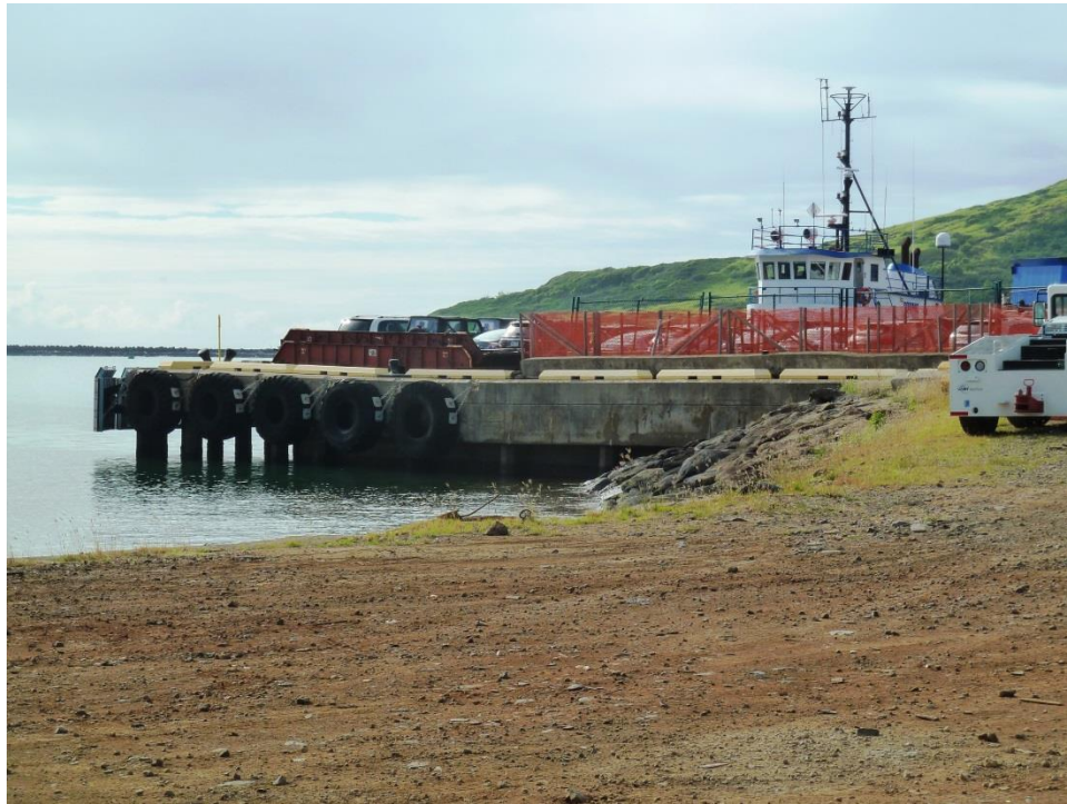
Figure 4-7: Edge of Pier 3 showing closely spaced driven pile supports
