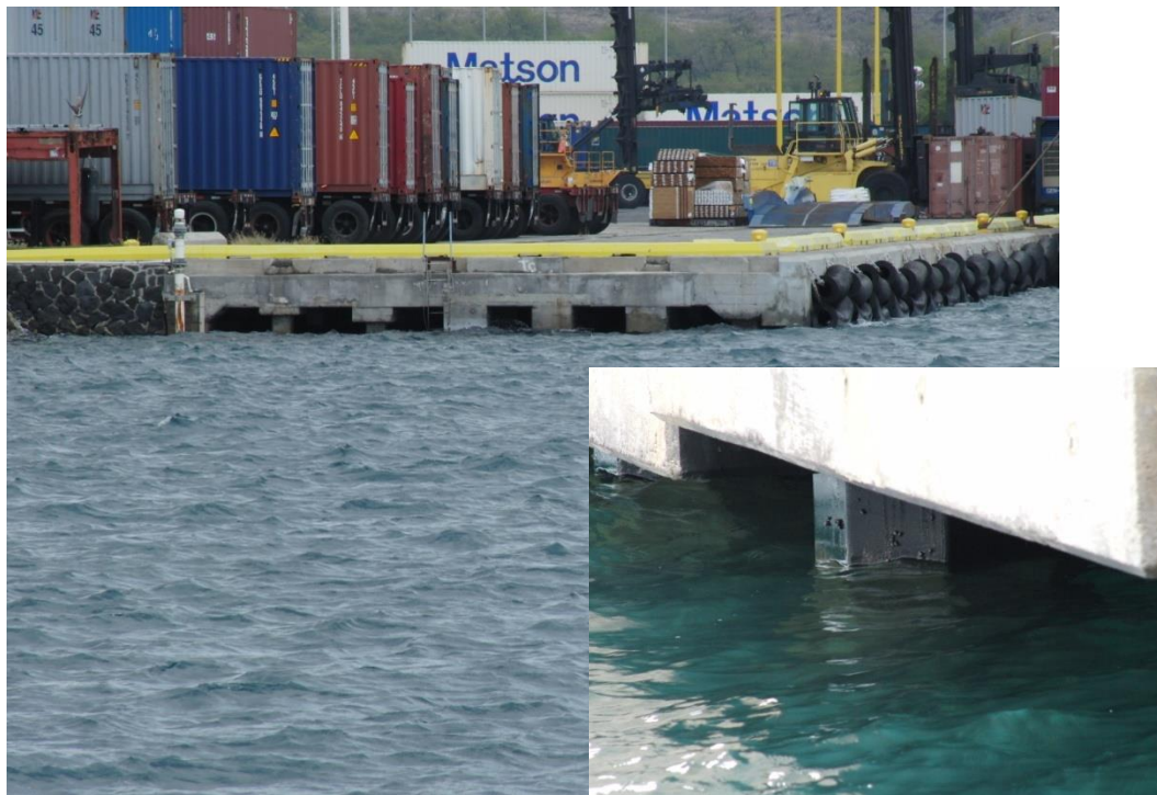
Figure 4-107: Pier 2 - concrete deck on piles (inset)
