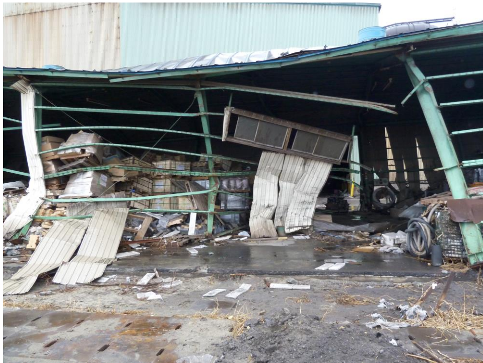
Figure 2-17: Damage to steel-framed warehouse in Sendai Harbor due to shipping container impact and damming effects
