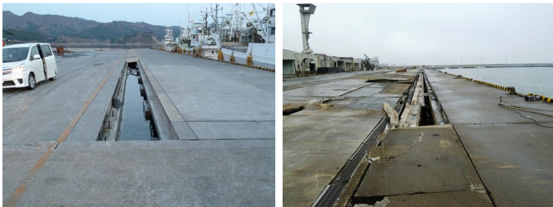
Figure 2-26: Concrete “breakaway” panels uplifted by the Tohoku Tsunami in Ofunato harbor (left) and Yuriagi harbor (right)
