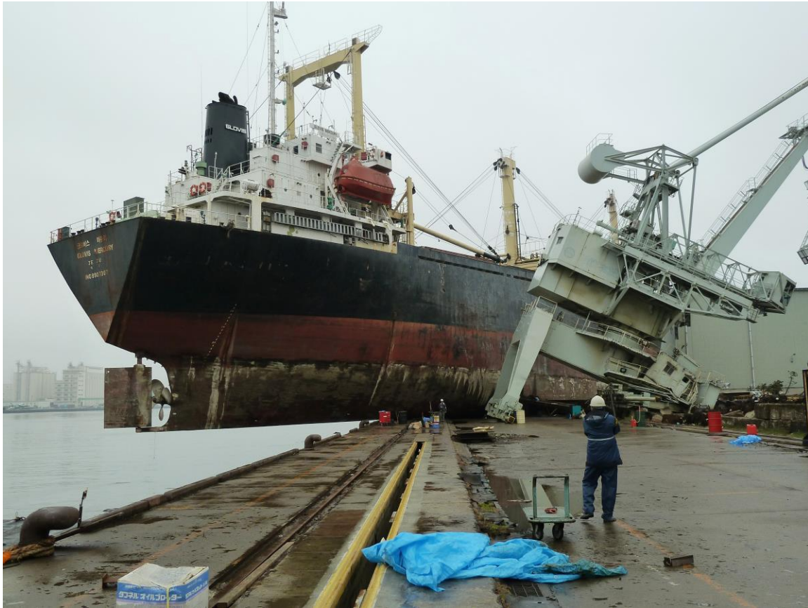
Figure 2-8: Ship impact damage to cargo crane in Sendai Harbor, Japan
