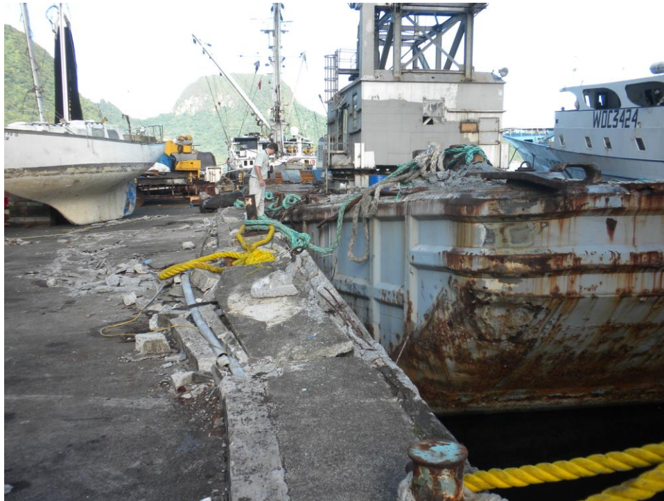
Figure 2-11: Barge uplift damage to concrete pier in Pago Pago Harbor, Samoa
