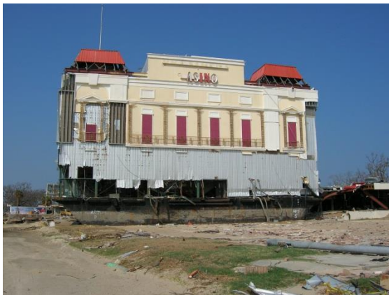
Figure 2-9: Barge-mounted casino that drifted over Highway US90 in Biloxi, Mississippi, destroying a number of structures.
