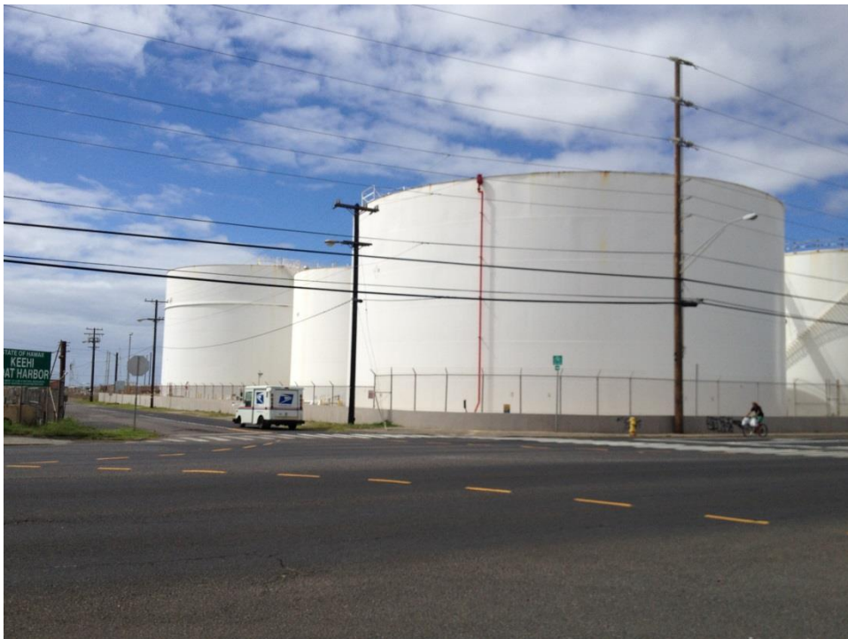
Figure 4-52: Aviation Fuel Storage tank farm with 3 ft. high containment wall
