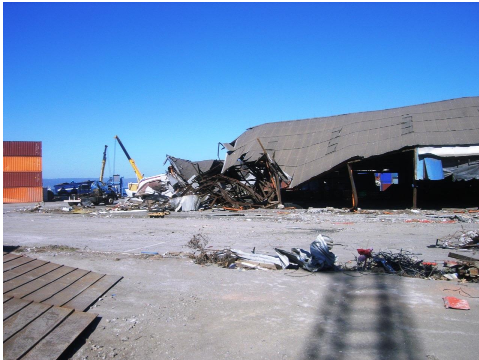
Figure 2-21: Damage to steel-framed warehouse due to shipping container impact and damming effects in Talcahuano Harbor, Chile.
