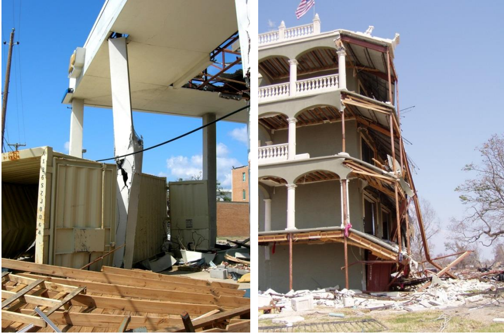
Figure 2-12: Structural damage to steel columns due to shipping container impact
