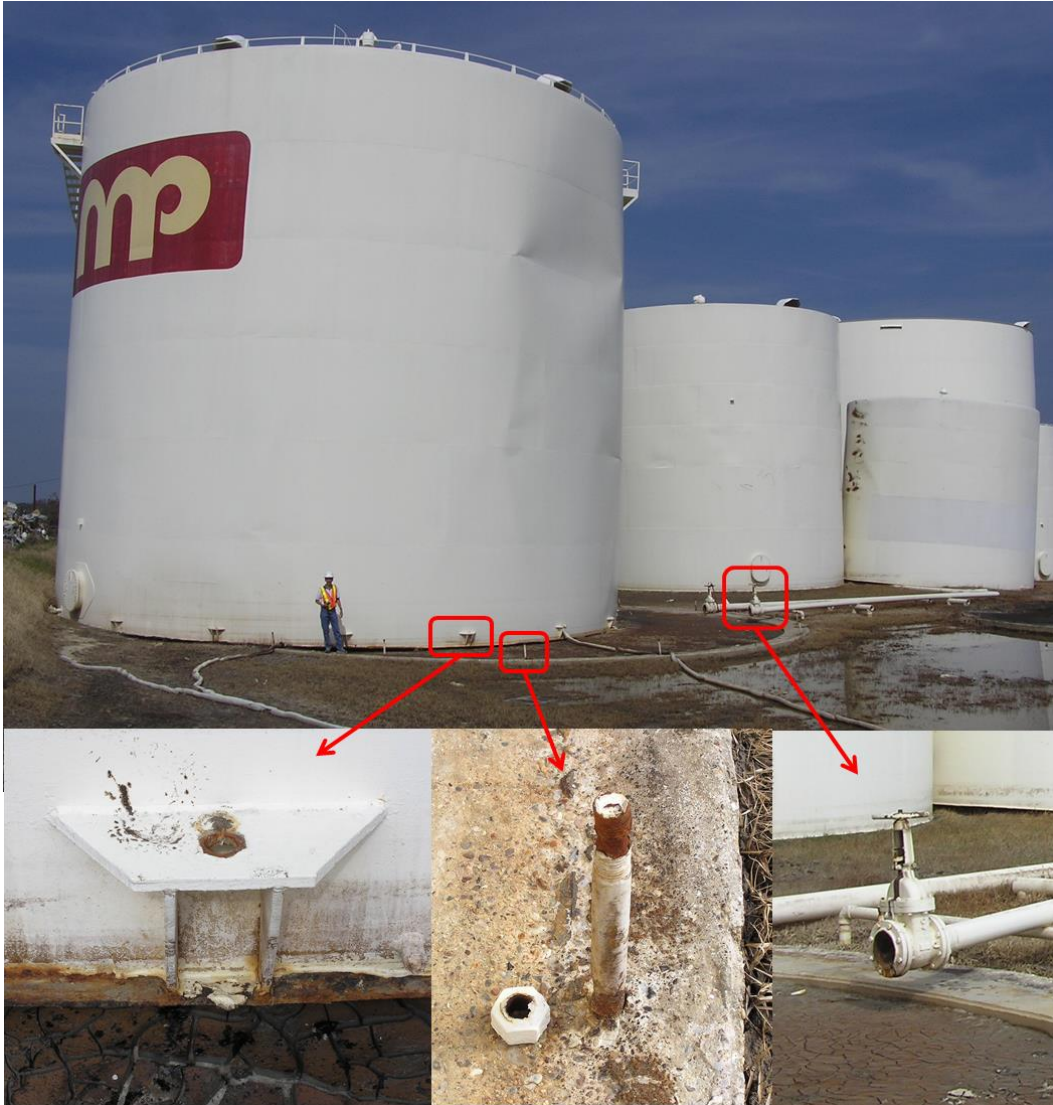
Figure 2-28: Fuel storage tanks floated off their foundations in Biloxi Back Bay, Mississippi
