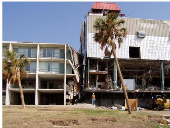
Figure 2-9: Barge-mounted casino that drifted over Highway US90 in Biloxi, Mississippi, destroying a number of structures.
