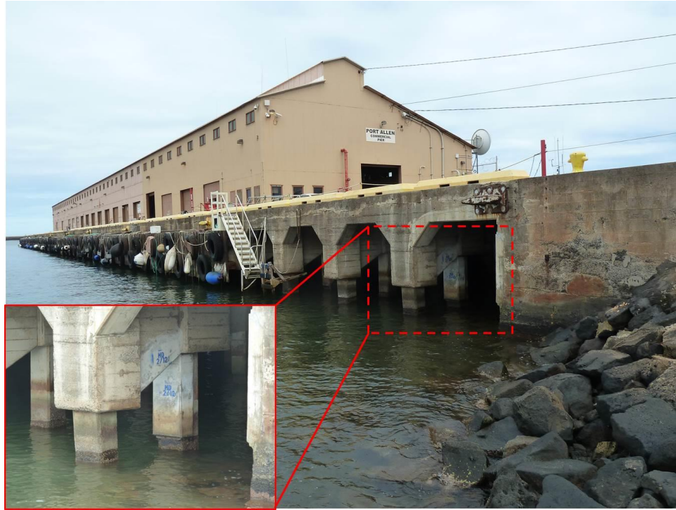
Figure 4-25: Pile supported pier and warehouse at Port Allen
