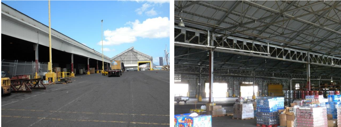
Figure 4-60: Steel framed warehouse on Piers 31 to 33
