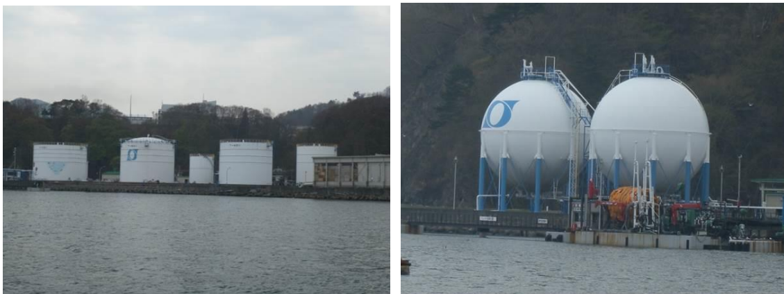
Figure 2-32: Undamaged fuel tanks (left) and LNG tanks (right) at Kamaishi Harbor after the Tohoku Tsunami
