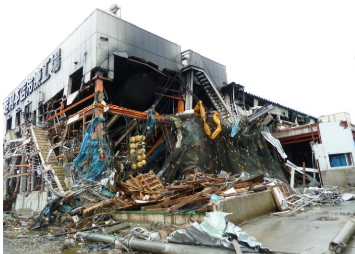
Figure 2-38: Port buildings with intact structural elements but extensive cladding damage; Kesennuma (left) and Taro (right)
