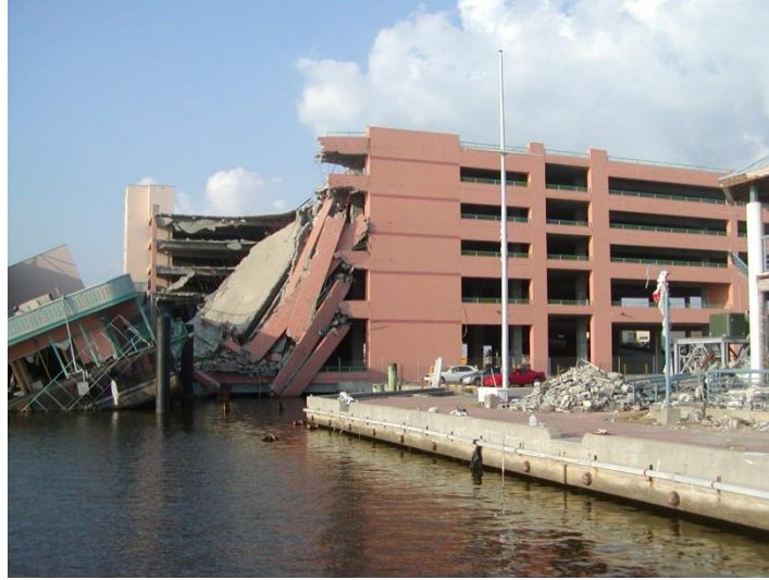
Figure 2-10: Partial collapse of prestressed concrete parking structure due to impact from barge moored adjacent to the structure
