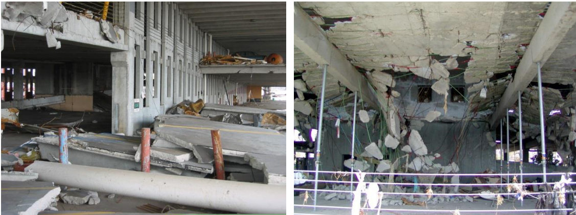
Figure 2-23: Damage to precast parking structure in Gulfport (left) and prestressed cast-in-place parking structure in Biloxi due to hydrostatic and hydrodynamic uplift
