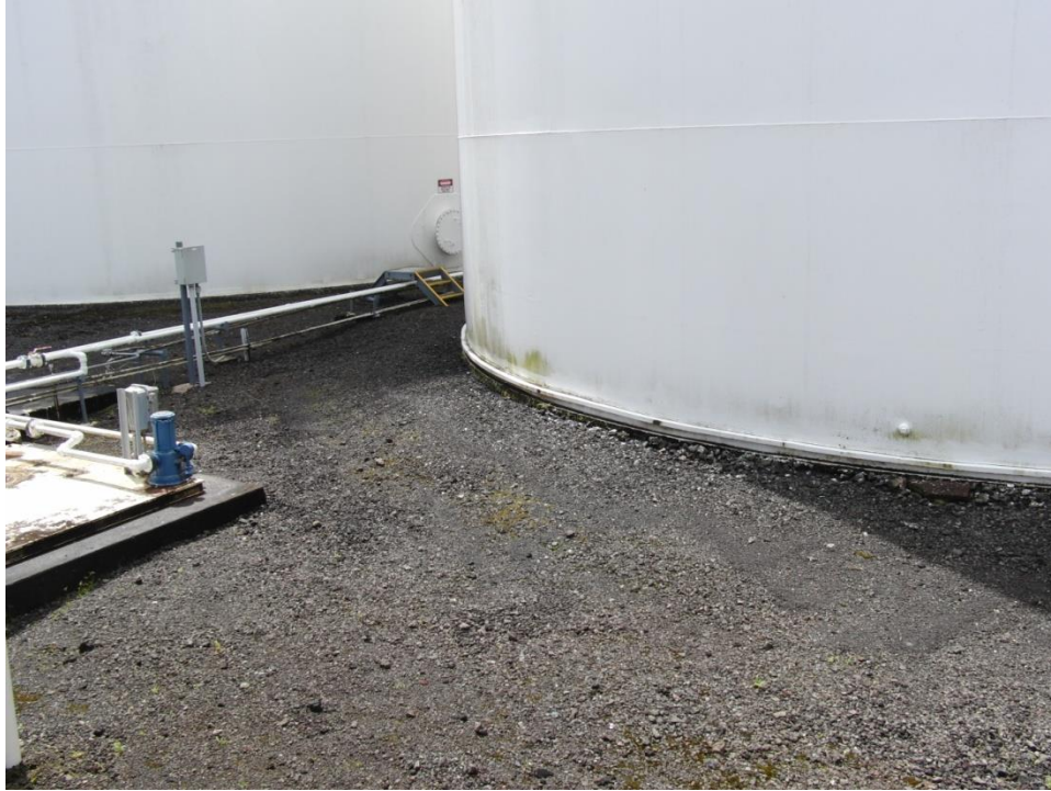
Figure 4-100: Tank bases resting on concrete slab without uplift restraint
