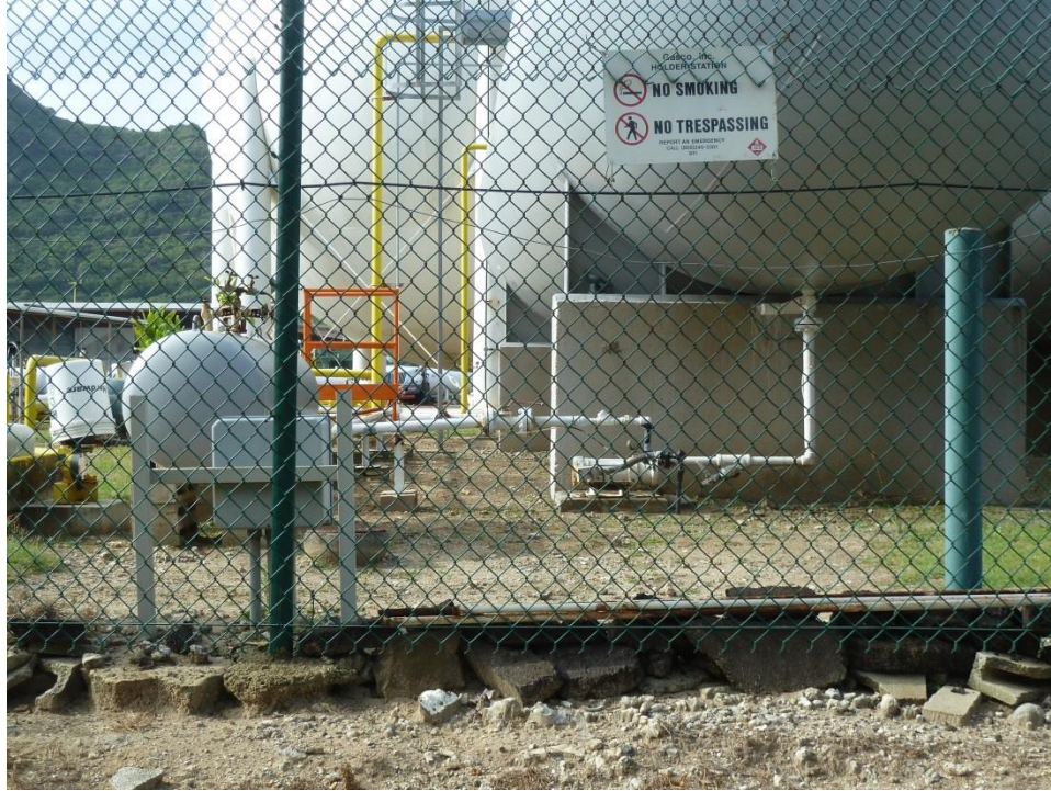
Figure 4-15: Gas tank connection to concrete foundation.
