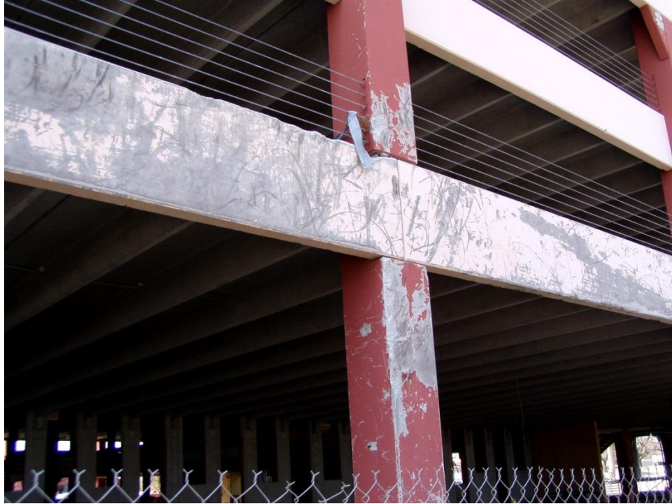
Figure 2-43: Superficial impact damage to parking garage beams and columns at Gulfport Harbor, Mississippi
