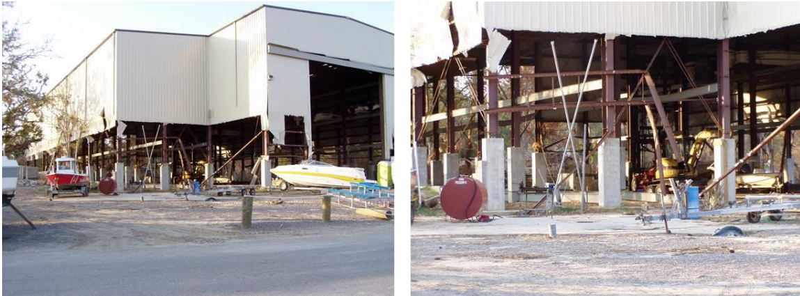
Figure 2-35: Damage to light sheet metal cladding on steel framed warehouse in Ocean Springs, Mississippi
