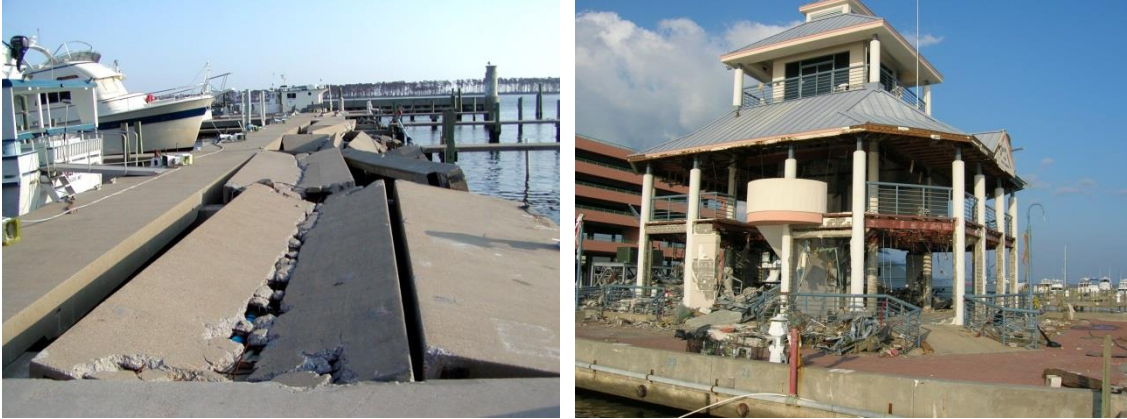
Figure 2-22: Hydrodynamic loading damage to concrete pier and steel harbor building at Joint Cadet Marina in Biloxi, Mississippi
