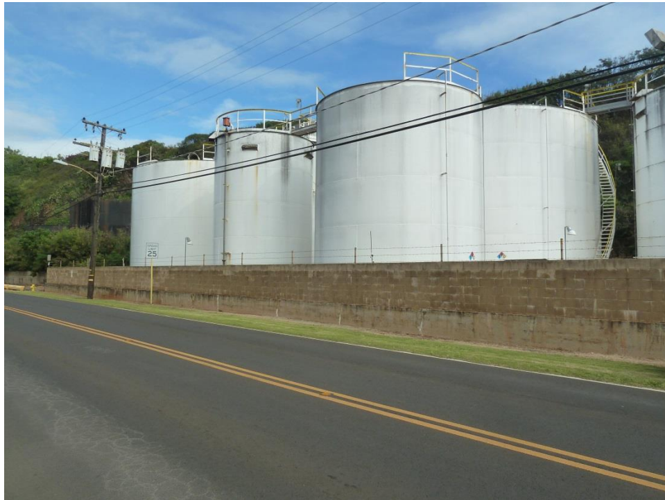
Figure 4-12: Containment wall around Aloha fuel storage facility at Nawiliwili Harbor
